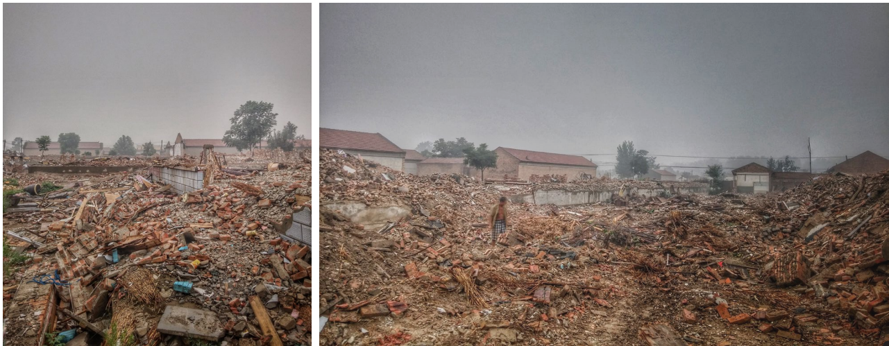
Fig 4.6. Villages Currently Under Demolition
