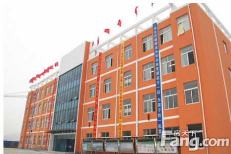
Fig 4.9. 21st Central Primary School - Reflective of a Urban School Type With a Multi-Story Block Building.
