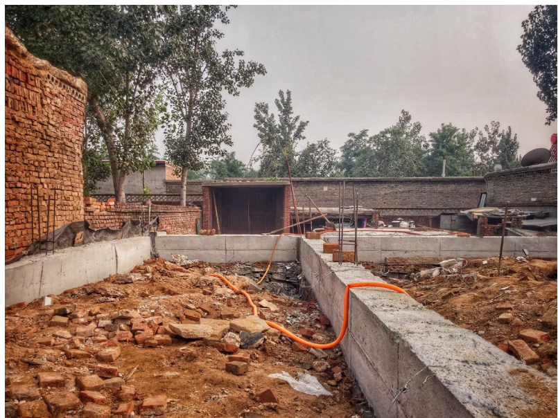
Fig 2.16. House Under Construction
