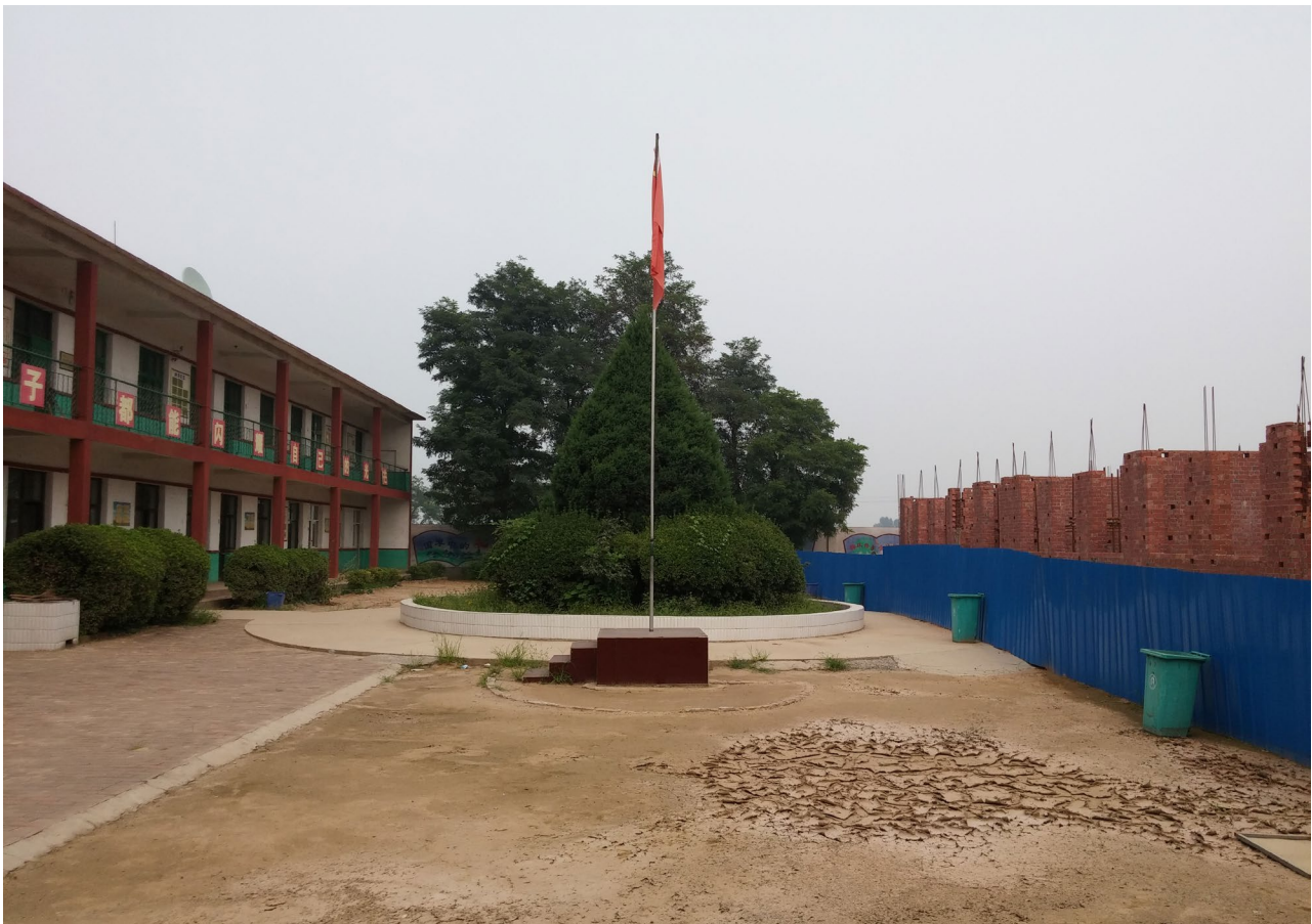
Fig 2.20. New School Under construction
