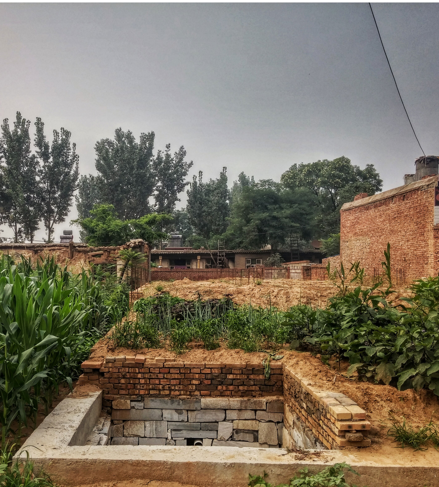
Fig 3.26. Abandoned Construction in Baodi, Hebei.
