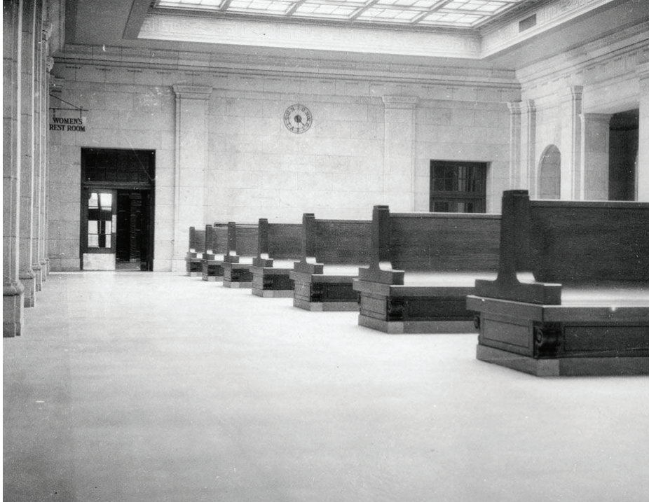
Figure 2.11 West Wing waiting room at time of opening. Early 1930s
