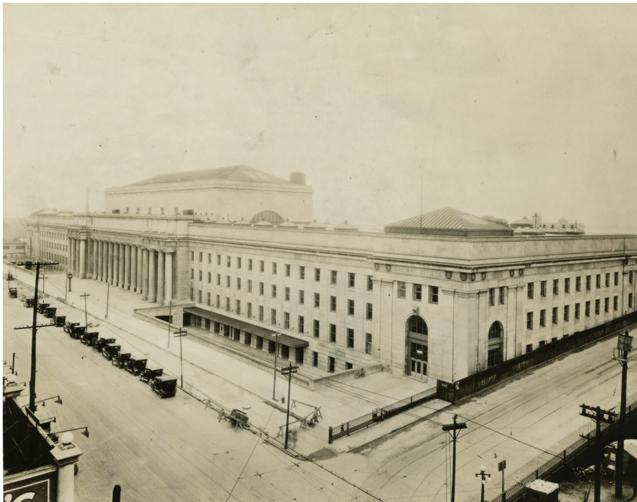
Figure 1.9 Recently completed Union Station.
