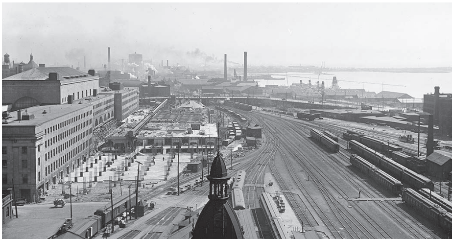
Figure 1.5 Union Station under construction. 1927
