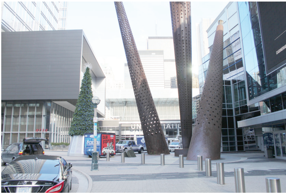
Figure 1.30 Union Station south entrance nearing completion. 2016
