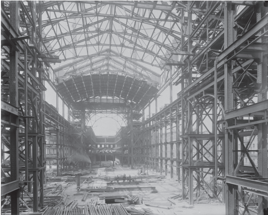
Figure 1.7 Union Station under construction, 1916
