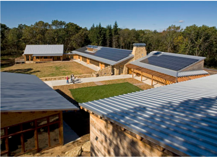
Fig. 1.2 Aldo Leopold Centre Carbon-Neutral Building Baraboo WI, USA
