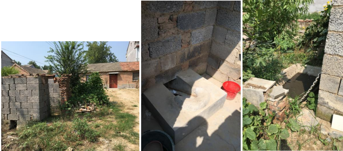
Figure 3.4 (a) Typical location of sanitation facility (b) Pour flush using bucket pit latrine (c) Manure from human feces
