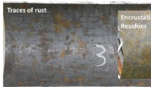
(c) Section 3 cleaned using rack-feed boring equipment.
