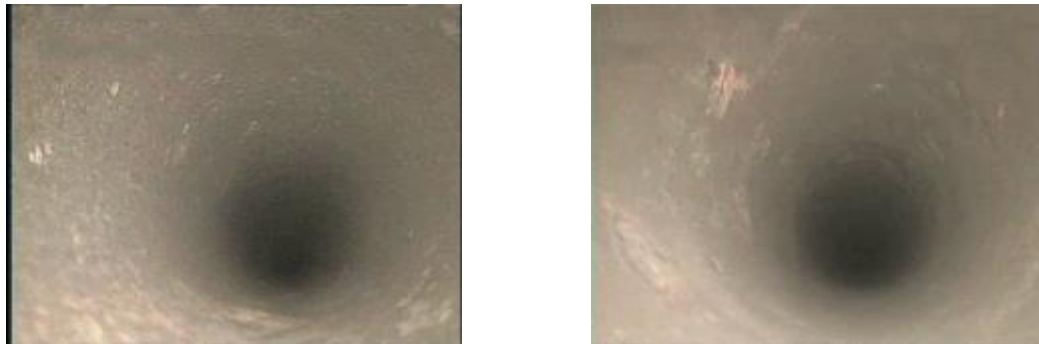
(b) Albert Street pipe after cleaning.
