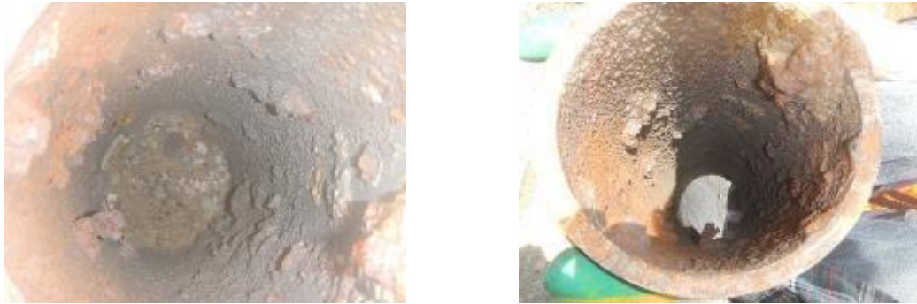
(a) Albert Street pipe before cleaning.
