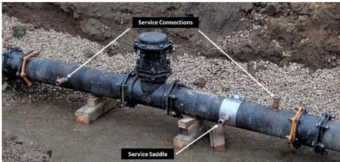
Figure 3.13: Spool with service connections and service saddle.
