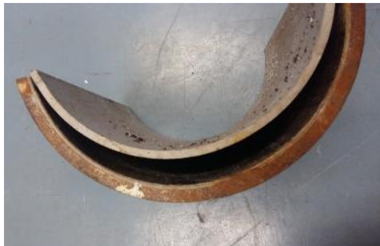
Figure 3.28: Pipe section with no lining adhesion with the host pipe as liner separated after jet cutting
