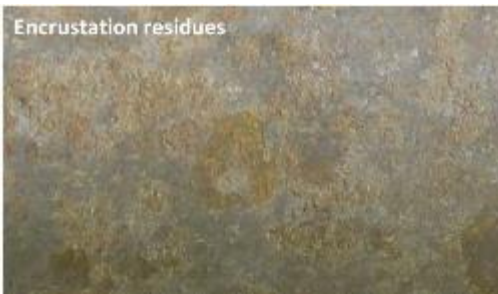
(c) Section 3 cleaned using rack-feed boring equipment.
