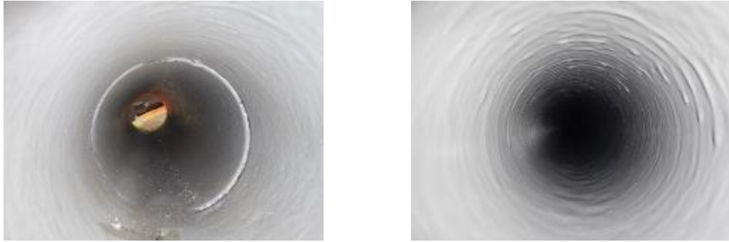
Figure 2.8: Albert Street pipe after Lining.
