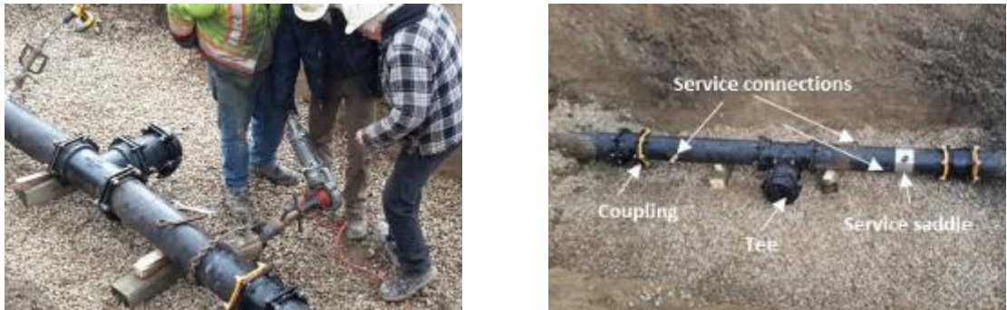
Figure 3.3: Installation of pipe spools with connections, tees and couplings.
