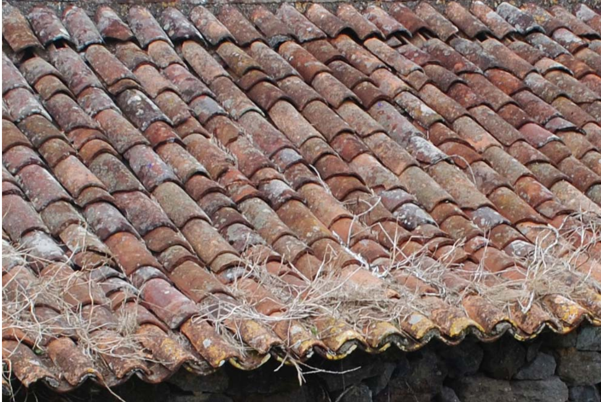
Fig. 1.66. Tiled roof with local tiles
