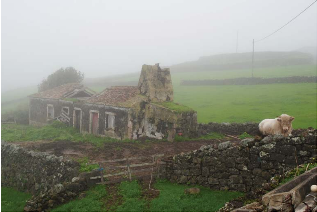
Fig. 1.28. Vacant house in Santa Bárbara, Terceira
