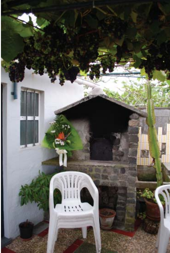
Fig. 1.86. Contemporary exterior wood oven
