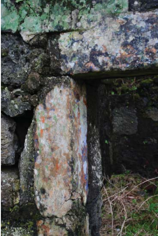
Fig. 1.75. Door frame showing layers of paint
