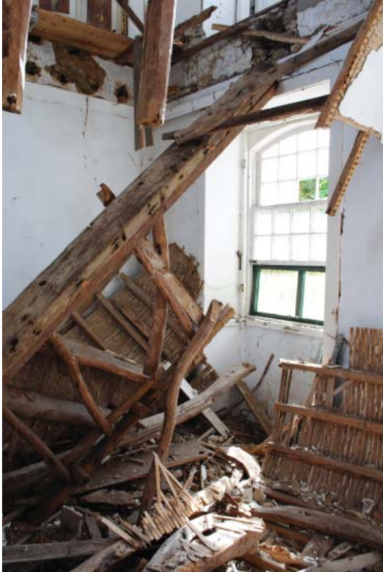
Fig. 1.71. Wooden floor beams and structure, and interior partitions
