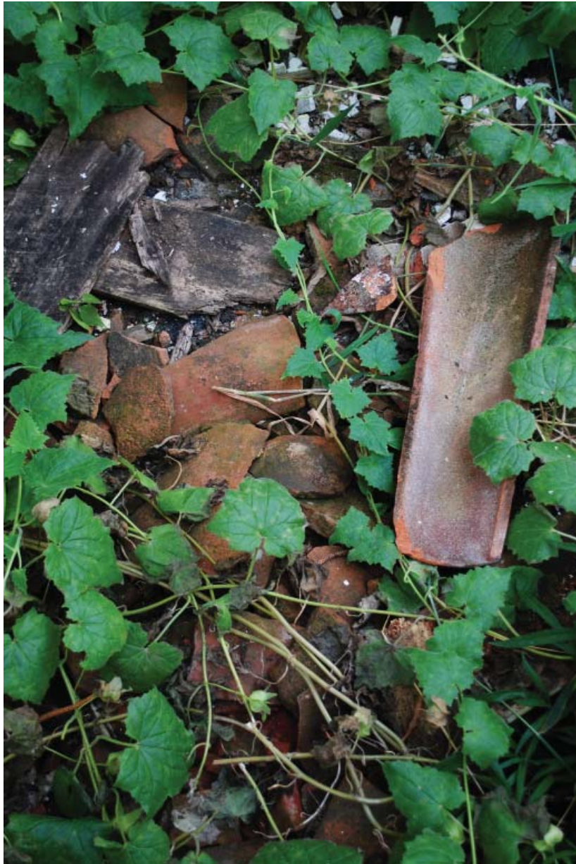
Fig. 1.44. Rubble and vegetation inside an abandoned house
