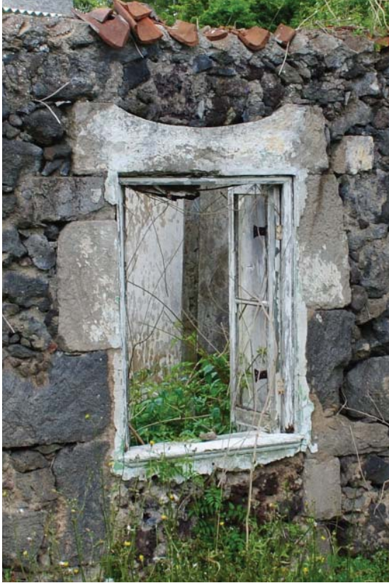
Fig. 1.63. Inverted lintel
