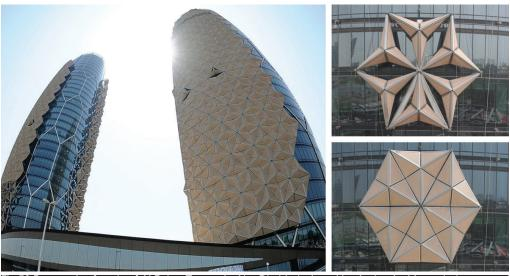
Fig.50 Responsive façade of Al Bahar Towers in Abu Dhabi, designed by Aedas Architects Ltd
