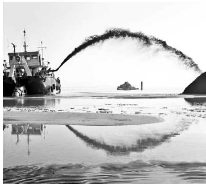
FIGURE 24 Dredging is a common technique used in landscape creation that is quite disruptive on the surrounding landscape. Sea floor disruption lifts loose sediment, lowering visibility and starving coral reefs, the loss of coral contributes to beach erosion, and the reaction continues.
