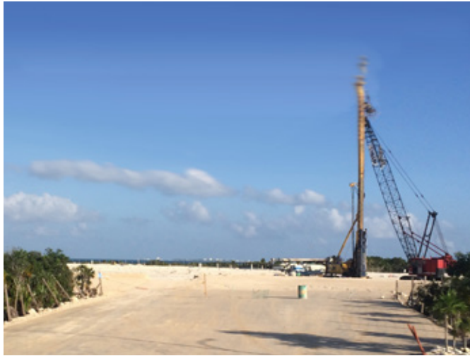
FIGURE 26 Beach front properties are cleared flat.
