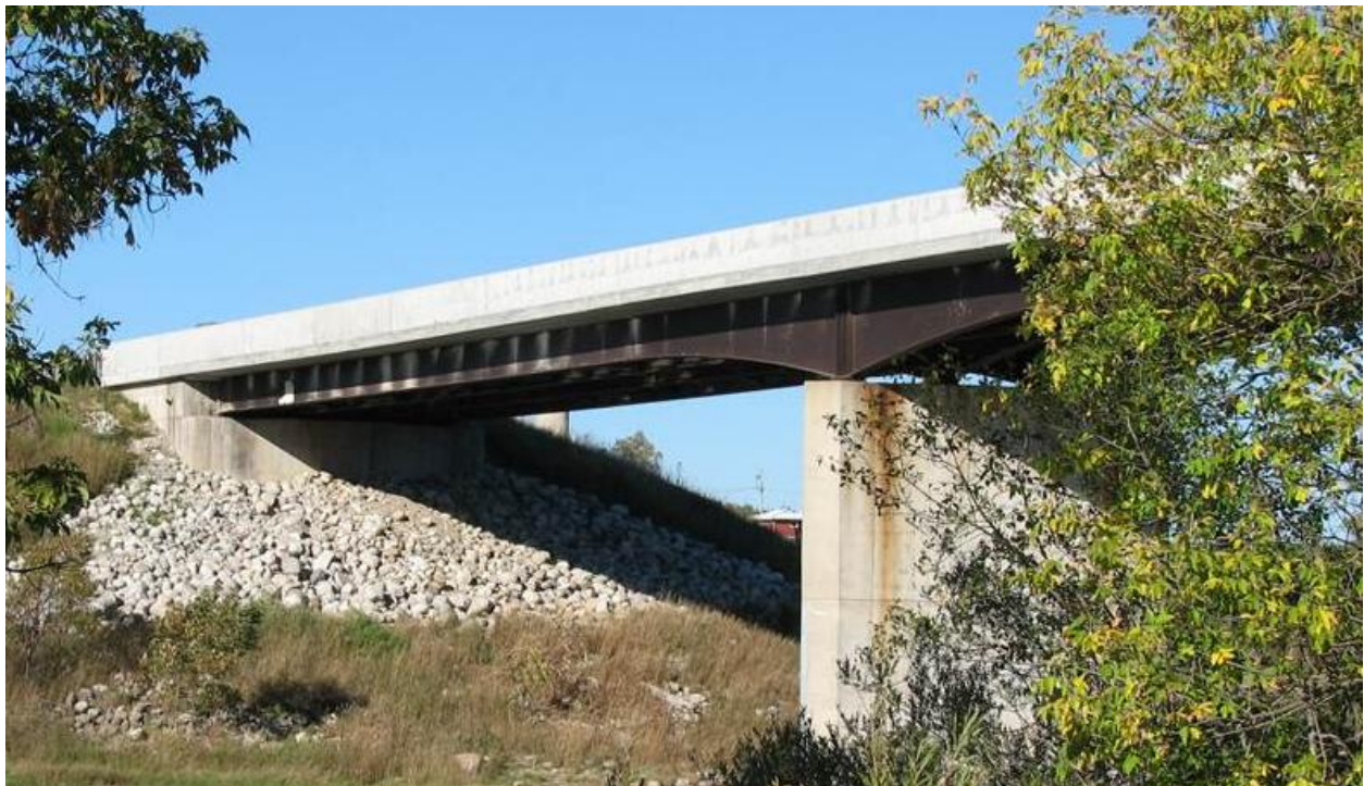
Figure 2-1: Steel-concrete composite bridge
