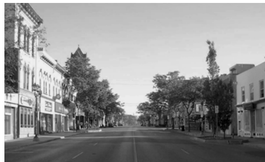
Fig. 166. King Street in Midtown in front of KCI Secondary School. The transition between the road and curb is abrupt.
