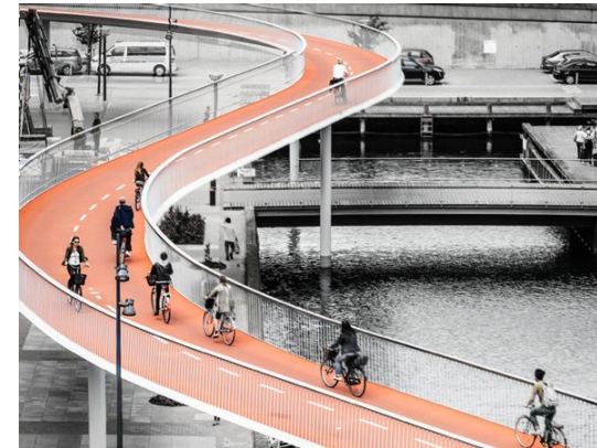
Fig 278. The Cykelslangen, or Cycle Snake is an elevated cycle path designed by Dissing and Weitling Architects for a busy pedestrian shopping area in Copenhagen. The path enables cyclists to pass through the area without having to haul their bikes up and down stairs, and frees the ground level for pedestrian traffic.
