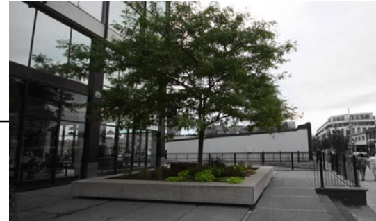
Fig 241. Above. Raised planter for trees and plantings, with perimeter bench atop podium. This type of planter provides additional soil and protection for the tree.
