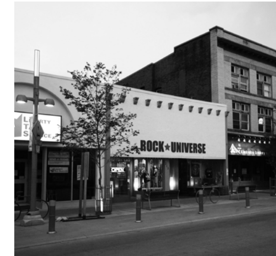
Fig. 230. Removable bollards positioned to the street side of parking space to close off portion of street from parked cars. This can be done if a business would like space in front of their business for cafe tables, or if extra bike parking is needed on site.
