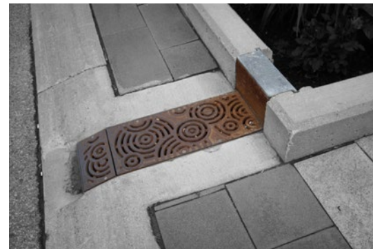
Fig. 259. Storm water grate feature in Downtown Kitchener. When there is rainfall, water is directed into the planting beds, where it absorbs into the soil and helps to water the trees and plants. If there is extreme rainfall, runoff water overflows into the storm drain to prevent flooding.
