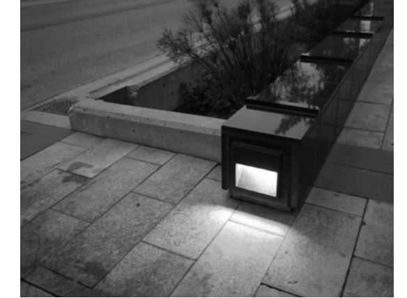
Fig 245. Above. Street lighting in Downtown Kitchener. The integration of low lighting in planting beds brightens the sidewalk and provides ambient lighting.
