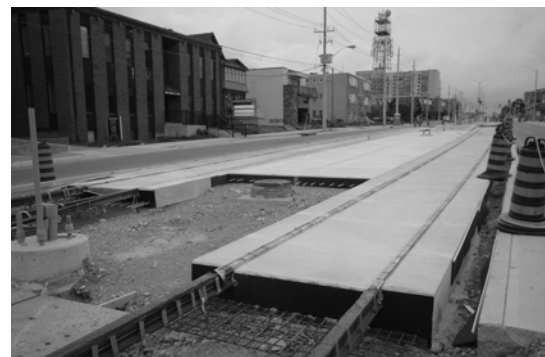
Fig 252. Pavement of LRT track at College and Spadina in Toronto.
