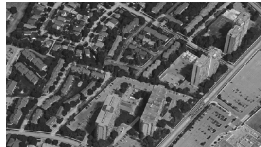
Fig. 213. Towers in the park adjacent to Fairview Mall in Kitchener. The only amenity local to this neighbourhood is Fairview Mall, which only provides big box retail stores. This scenario is better than some, where the towers are surrounded only by other homes.
