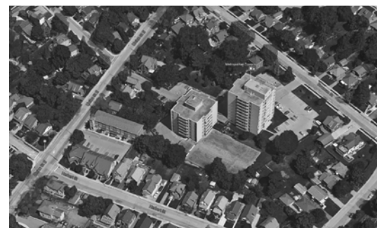
Fig. 214. Towers North of Mount Hope Cemetery in Kitchener. Surrounded by large parking lots and single detached homes, it would be a minimum 15 minute walk from the lobby of one of these towers to any sort of public amenity or retail establishment. This makes transportation difficult for local apartment dwellers to have access to daily amenities without the use of a car, or very frequent and reliable public transit. With many apartment buildings charging a monthly fee for parking on-site, this adds a level of expense to a housing option that many people seek for its level of affordability.
