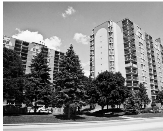
Fig 121. The Gresham Place apartments at 600 Greenfield Avenue. The towers are located near Fairview Park Mall and the Conestoga Parkway. They contain private building amenities, but no ground floor public space. Although at a slight advantage being close to the mall, the buildings are still surrounded by a largely unwalkable site.
