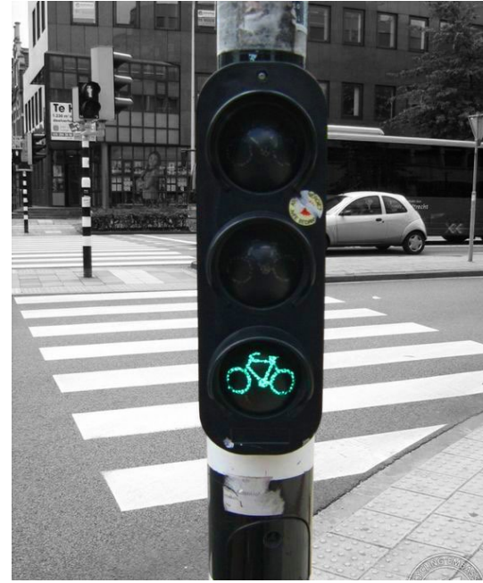
Fig 281. Bicycle traffic lights installed at eye-level to direct bicycle traffic flow in Amersfoort, Netherlands.
