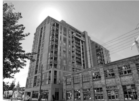
Fig 360. Top left. Bauer Loft Condo Building 15-storey tower and neighbouring historic redevelopment.
