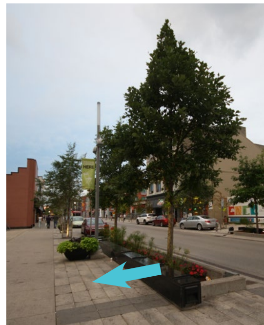
Fig. 260. Seams between granite pavers also allow water to percolate through into the soil below, reducing the reliance on storm sewers.
