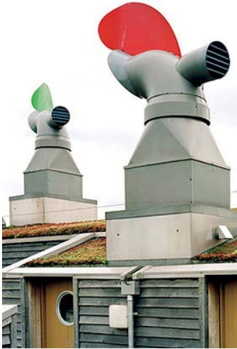
FIG. 7 BEDZED WINDCOWLS Image shows the windcowls used within the BedZED development to passively cool interior spaces. Image retrieved from: Andrews, Kate. Digital image. Inhabitat. January 17, 2008. Accessed December 26, 2017. https://inhabitat.com/bedzed-beddington-zero-energy-development-london/ .
