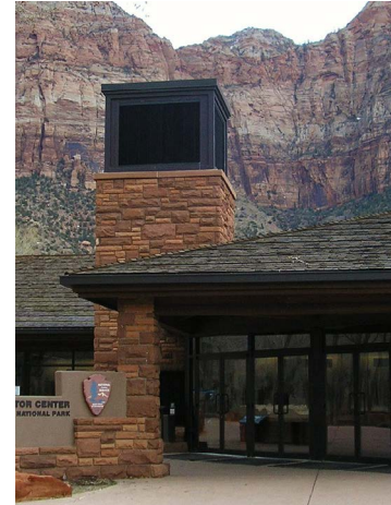
FIG. 9 ZION NATIONAL PARK VISITORS CENTRE Image of the cooltowers used to passively ventilate the interior of the Zion National Park Visitors Centre. Image retrieved from: Johnson, Bruce. "Zion National Park - Visitor Center." Digital image. Flickrriver. March 20, 2006. Accessed December 26, 2017. http://www.flickrriver.com/photos/alltheparks/2142498569/ .
