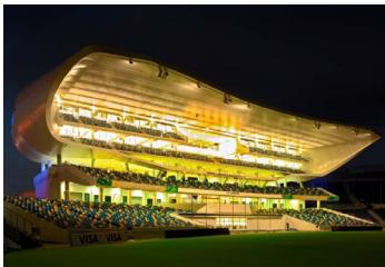
FIG. 8 KENSINGTON OVAL Image shows the formal design of the Worrell, Weekes, and Walcott stand at the Kensington Oval allowing for passive ventilation across the tiered stands. Image retrieved from: Richters, Christian. Digital image. ARUP Associates. 2007. Accessed December 26, 2017. http://www.arupassociates.com/en/projects/kensington-oval-barbados/ .
