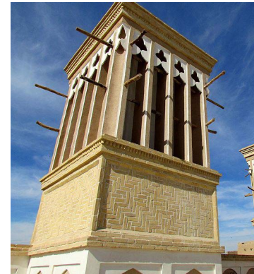
FIG. 4 TRADITIONAL WINDCATCHER Image shows the traditional design of a multi-directional windcatcher located in Dubai. Image retrieved from: Javaheri, Alireza . Digital image. 99% Invisible . Accessed December 26, 2017. https://99percentinvisible.org/article/windcatchers/ .
