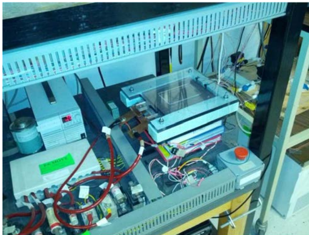
Figure 1. Experimental setup showing the battery and cold plates.
