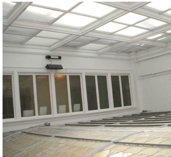
Figure 14 - Overlooking the Stained Glass Dome From the 2nd Floor
