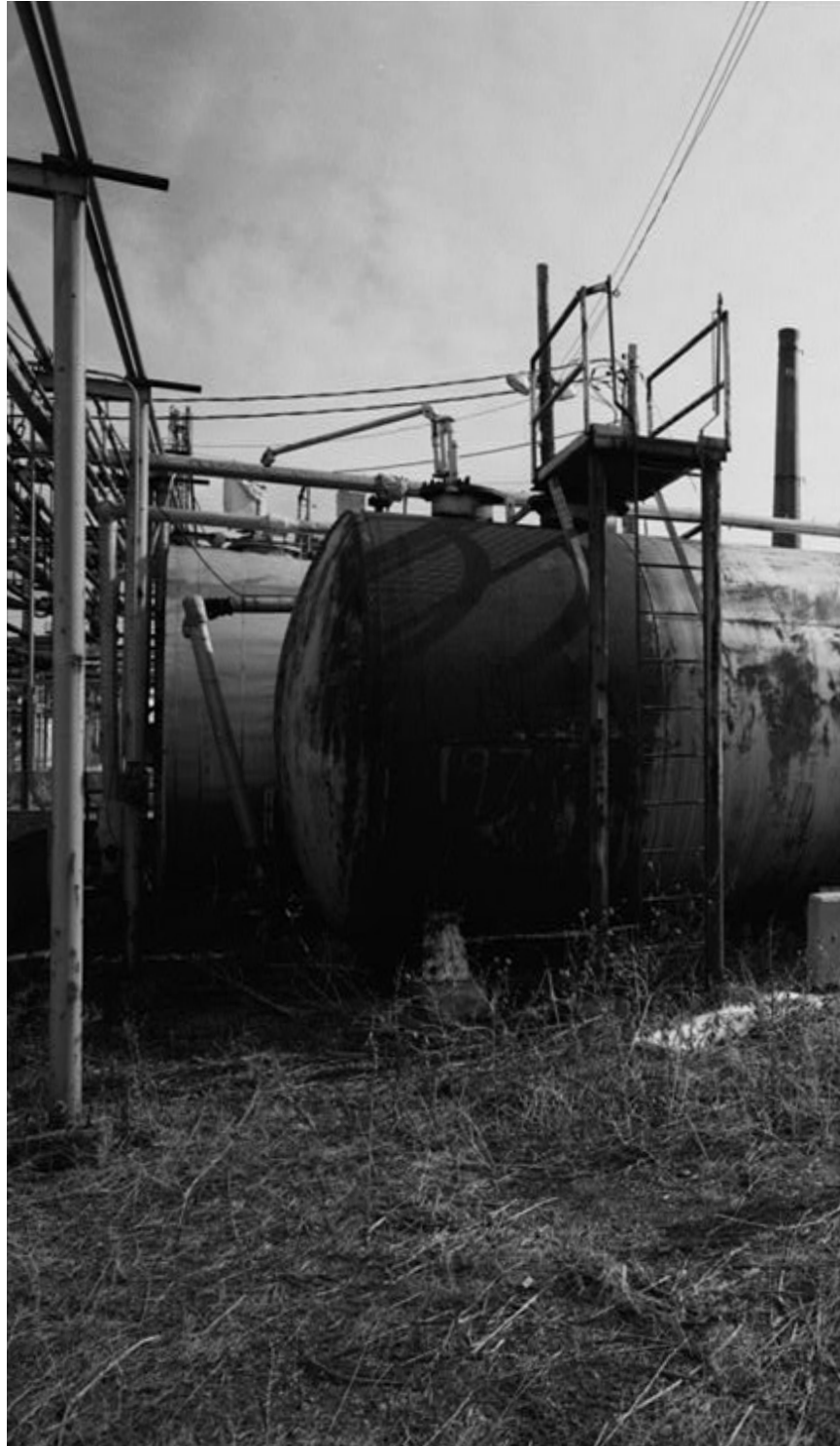
figure 2.73 Historic American Engineering Record, Creator, Rocky Mountain Arsenal, Storage Tank, December Seventh Avenue & D Street, Commerce City, Adams County, CO, 1968.
