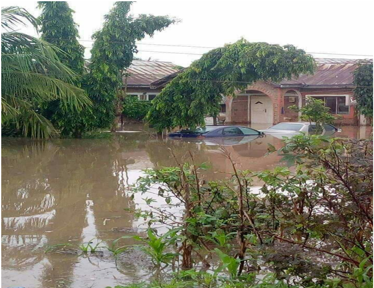
Figure 13: Flood Waters in Makurdi
