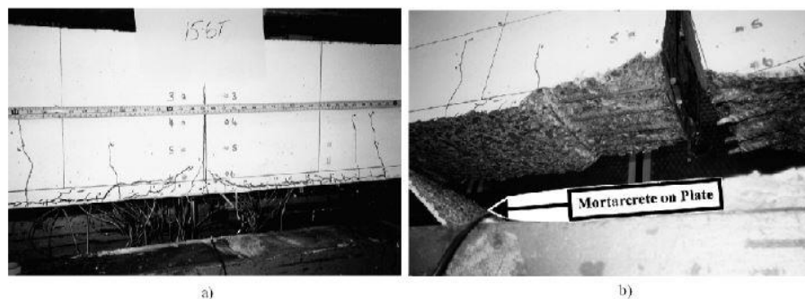
Figure 2.20: Debonding failure: (a) inclined cracks and concrete fracture near the midspan region; (b) the bottom of the beam at the midspan after failure (Sebastian, 2001)
