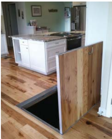
Attic trap door
