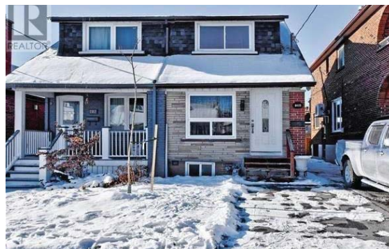
Fig. 2.13 Semi-detached house in York
