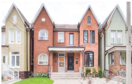
Fig. 2.12 Semi-detached house in Trinity Bellwoods
