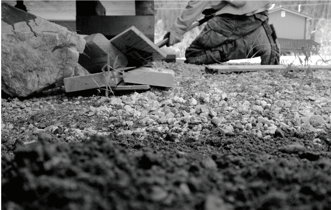
fig. 4.4 Detail of gravel fill and building materials
