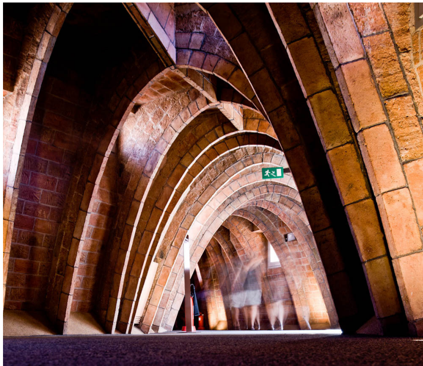
Figure 5.4 - (top) - Christopher Wren's sketch for a dome with a catenary profile Figure 5.5 - (bottom) - Antonio Gaudi's Casa Mila. Catenary curves are used as structural ribs
