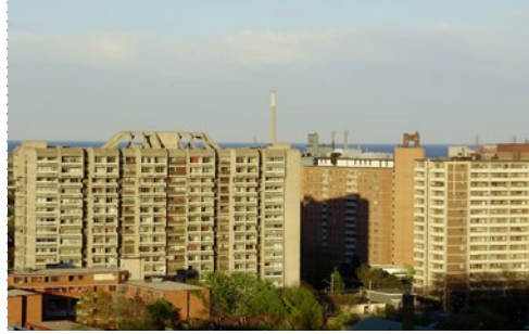
Moss Park houses were demolished to build Moss Park apartments.
