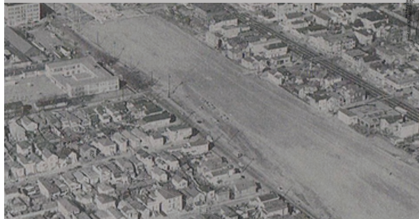
2. Fig. 1.26 Demolition for the construction of the Cypress Freeway
