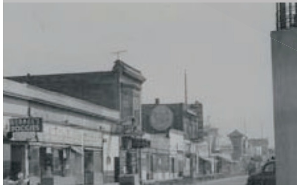
1. Fig. 1.27 Construction of BART tracks on 7th Ave.
