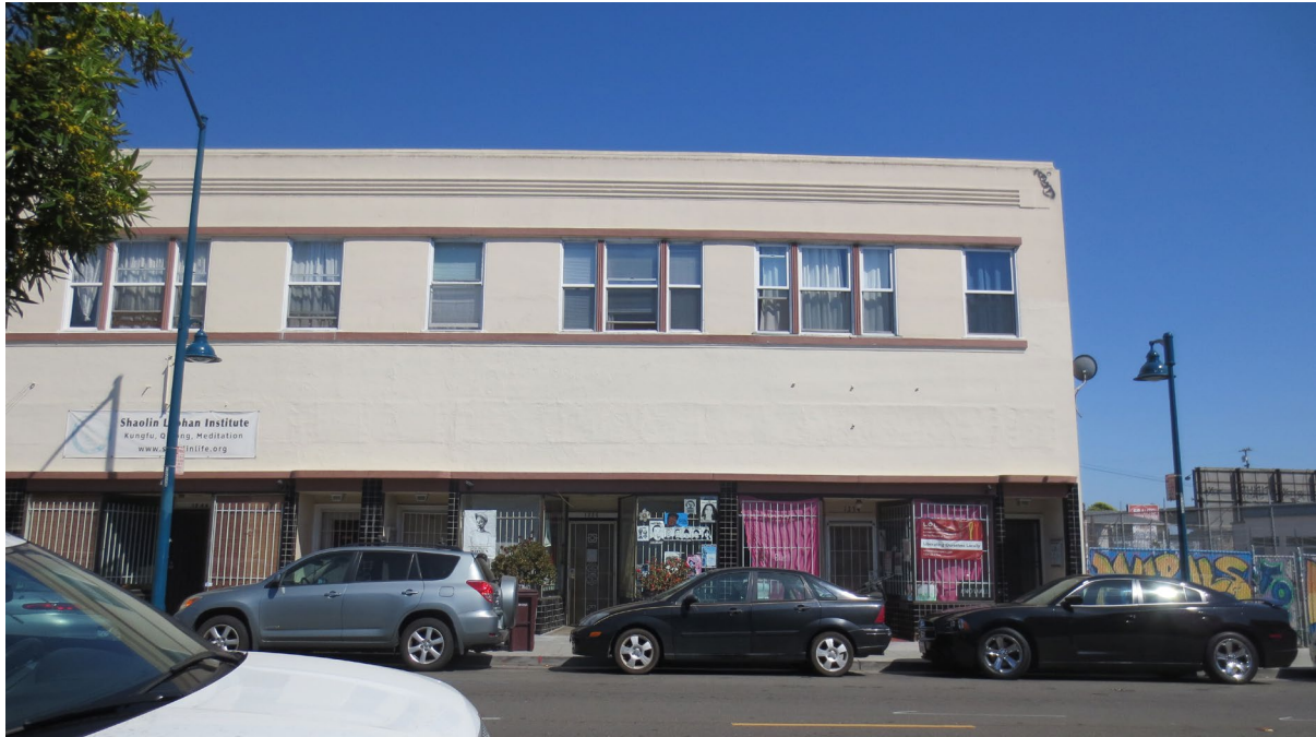
Fig. 3.15 23rd Ave. Building, front elevation
