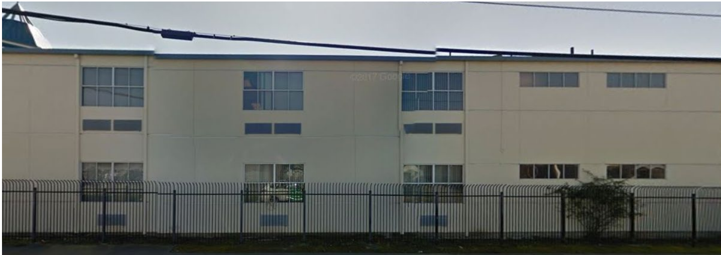
Fig. 1.34 Fencing at Allen Temple Baptist Church
