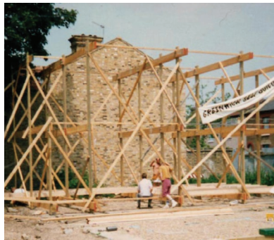
Fig. 4.10 Structural Scaffold: House framed using the Segal Method
