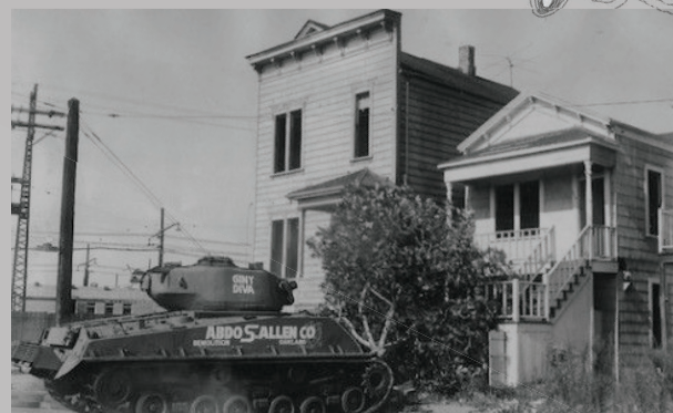
Fig. 1.28 Salvaged Sherman tank used for demolition in West Oakland, to make way for the construction of a USPS distribution centre
