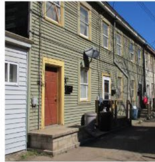
Nearby alley home
