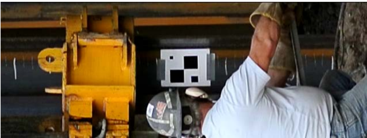
Figure 16 – Pile I-2 Raw Video Image with Obstruction Near the Target
