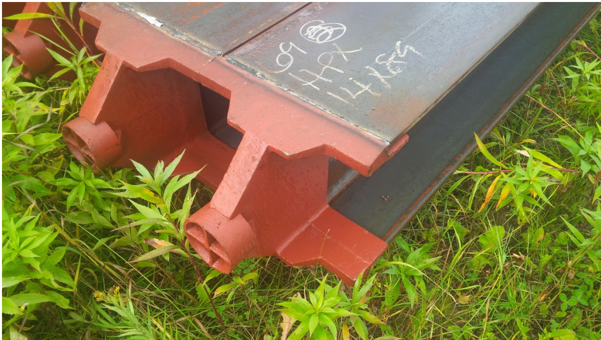
Figure 1 – Steel Pile HP 360x132 With Installed Titus Steel Rock Injector Point
