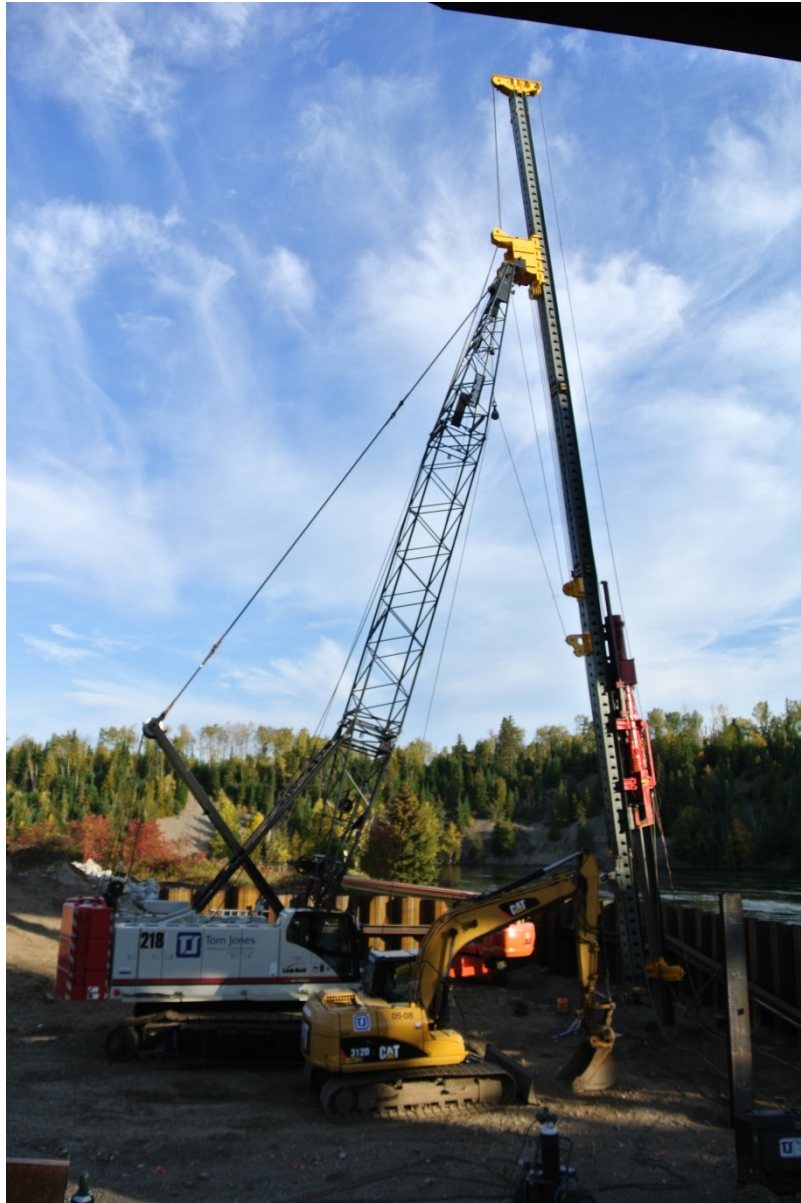
Figure 2 – Crane and Hammer
