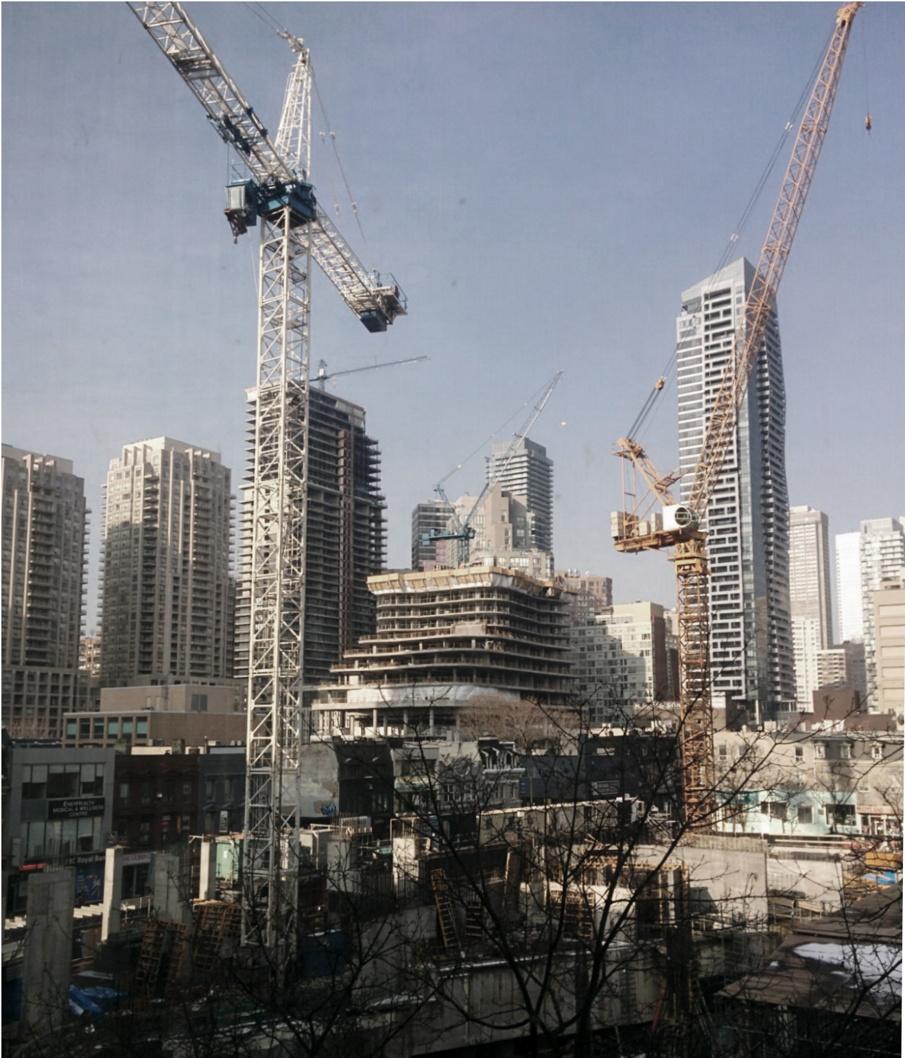
Fig. 1.1 Looking at construction from 475 Yonge Street towards Yonge Street.
