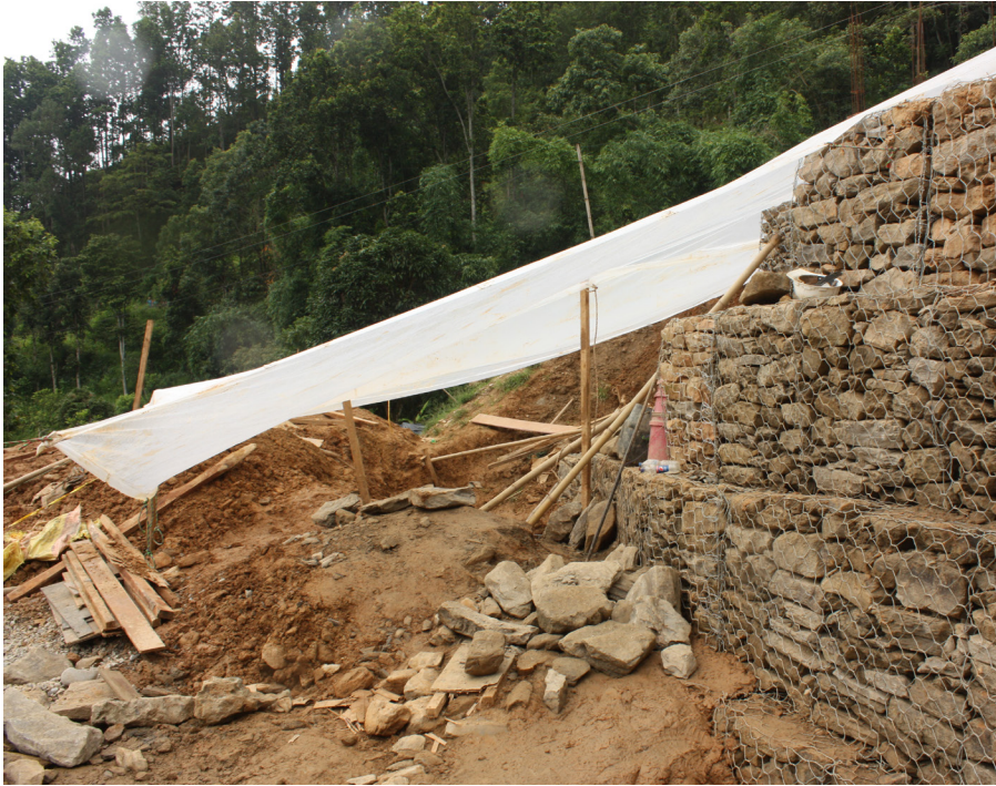
fig. 0.06 Construction of the gabion walls
