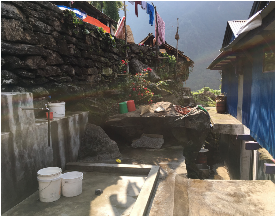
fig. 2.32 Public water tap, usually shared amongst numerous households
