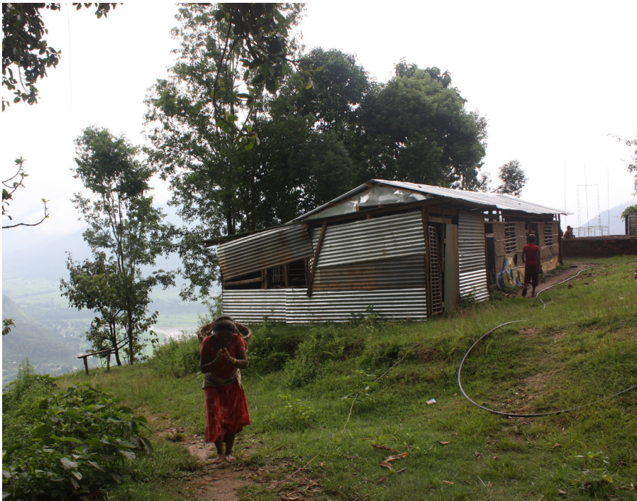
fig. 2.44 Temporary public school; in some regions children can be attending temporary schools for several years while permanent schools are being reconstructed
