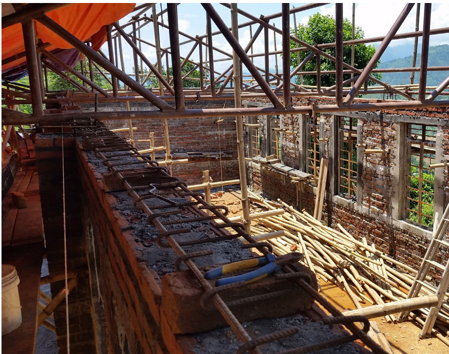
fig. 0.07 Tying rebar for the roof concrete band
