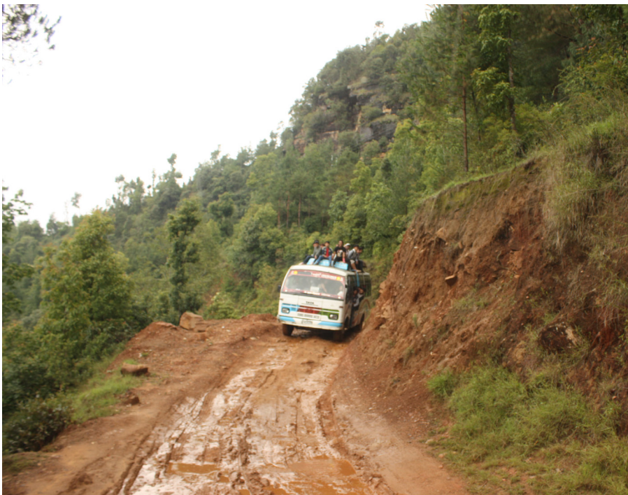
fig. 2.26 Smaller dirt roads connecting rural settlements to the highway; during monsoon season they often become inaccessible
