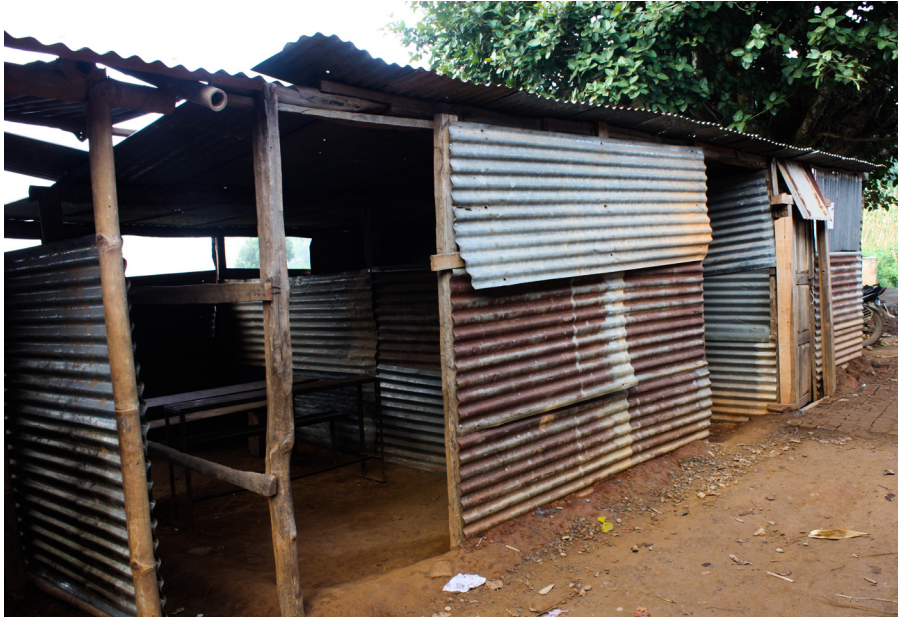
fig. 2.64 Temporary Learning Centre (TLC) in place of a public school that was damaged during the 2015 earthquake. At the time the photo was taken in August 2016, construction of a permanent school was just being completed.
