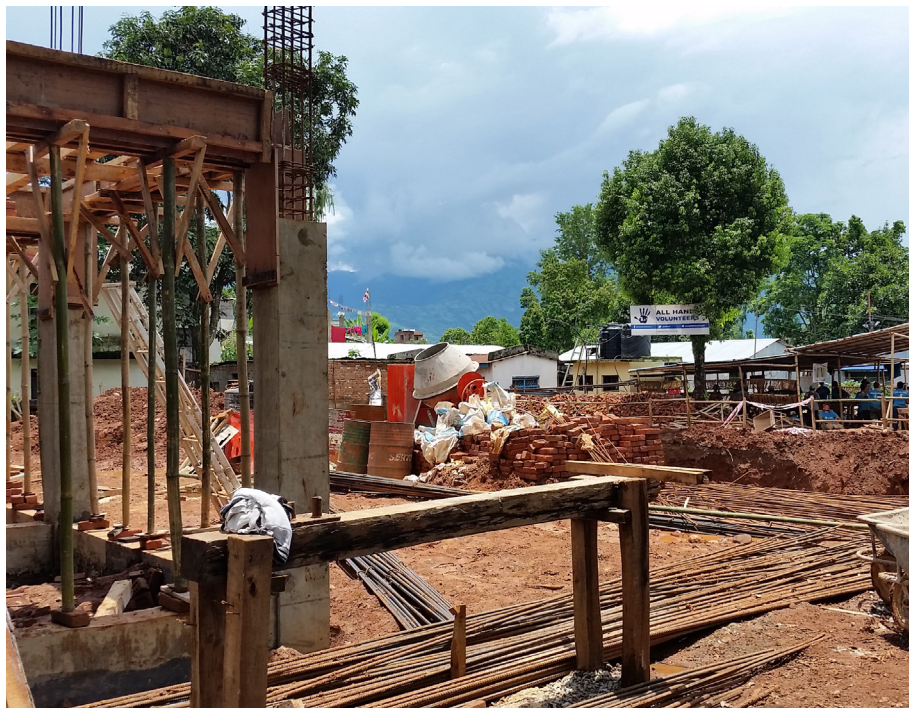
fig. 0.05 Excavating the foundations for the second school building on the site
