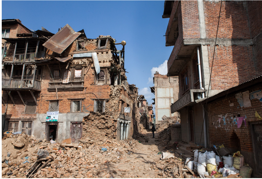
fig. 2.52 Damage from the earthquake. photo: ReSurge International
