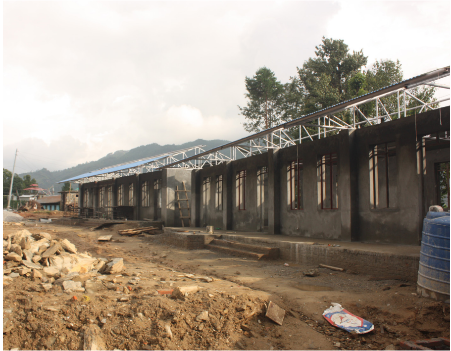
fig. 0.04 Sheets of corrugated metal installed over metal roof trusses
