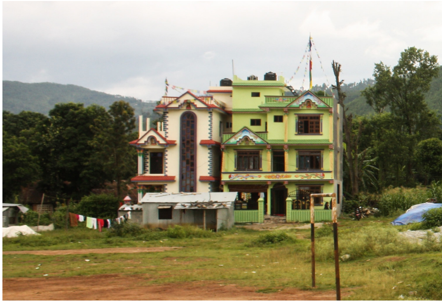
fig. 2.63 Private school in Trishuli, Nuwakot District
