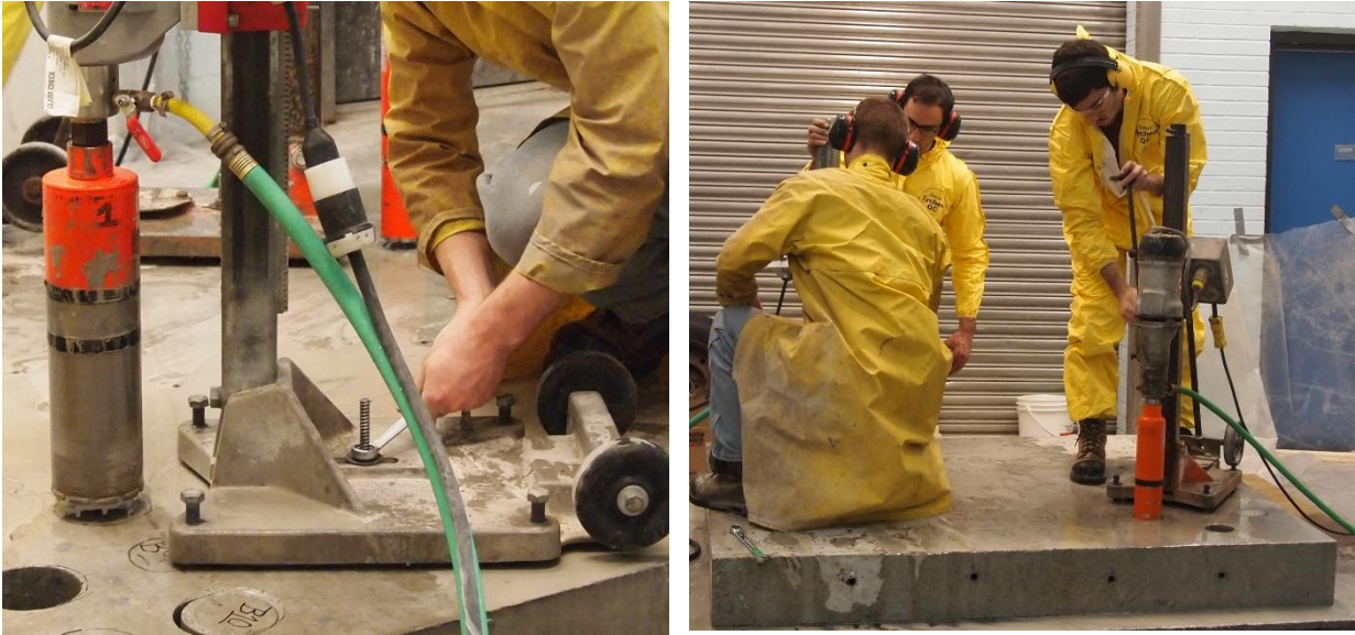
Figure 3.10 Anchored coring drill for coring of G1 girder webs
