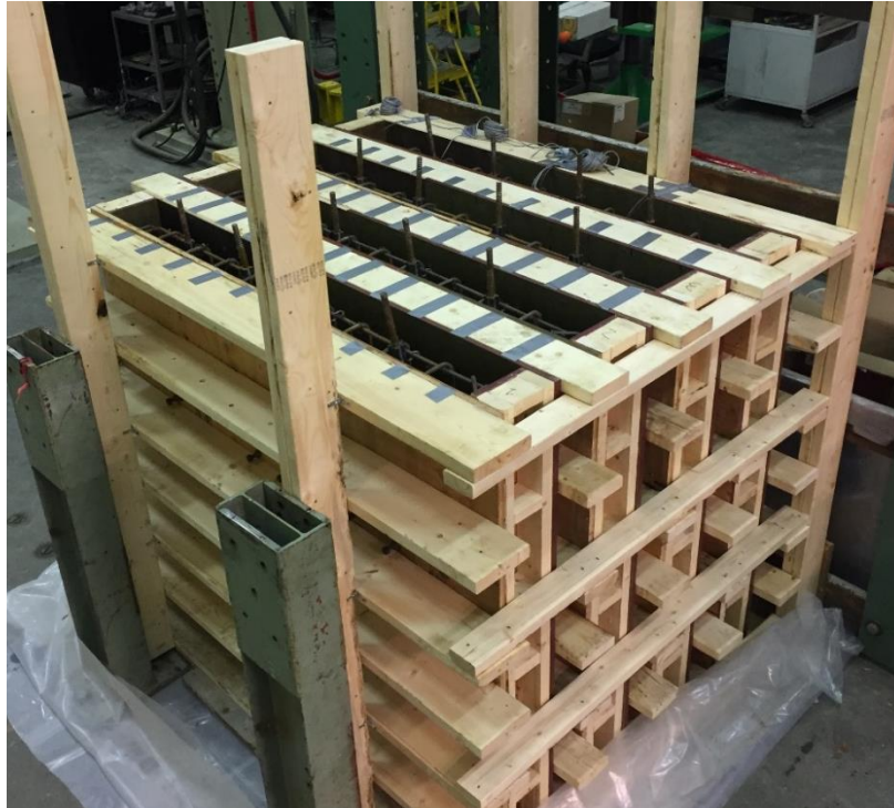
Figure 3.8 Constructed Formwork for G1 Girder Webs
