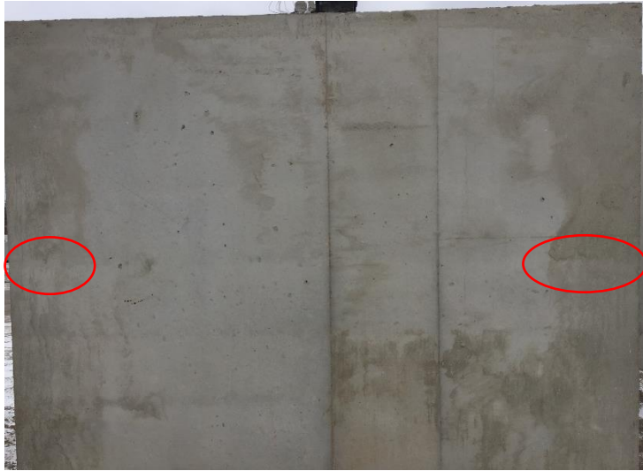
(a) Wall A – Pouring location
