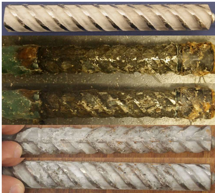
Figure C.48: 7.5-300 Batch – Corrosion Products on XM-28 AR 6.8. From top to bottom, a) original specimen, b) & c) corrosion products on the specimen upon removal from concrete, and d) & e) pitting corrosion identification on the pickled specimen
