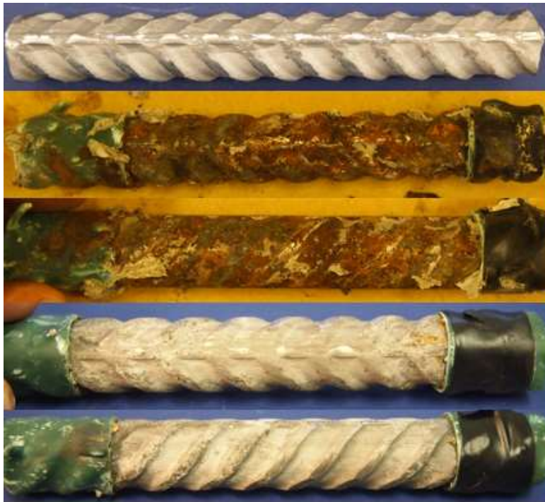
Figure C.71: 7.5-400 Batch – Corrosion Products on XM-28 AR 8.3. From top to bottom, a) original specimen, b) & c) corrosion products on the specimen upon removal from concrete, and d) & e) pitting corrosion identification on the pickled specimen
