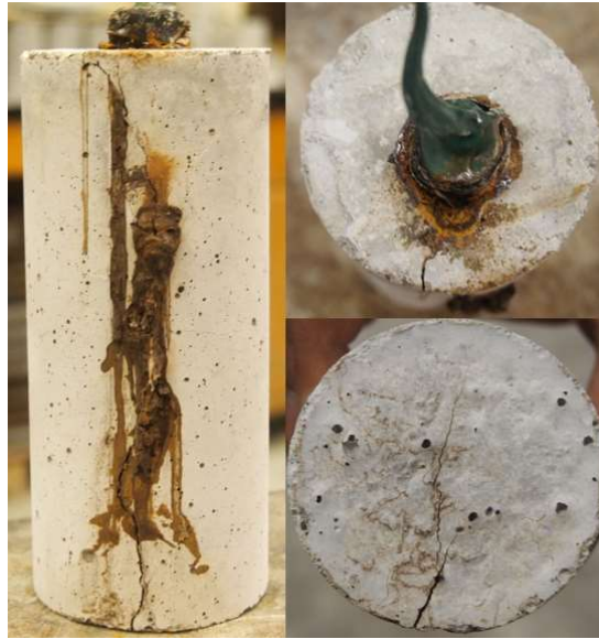
Figure C.60: RST 7.5-400 Batch – XM-28 AR 8.1 Corrosion Products causing Cracking of Concrete Specimen
