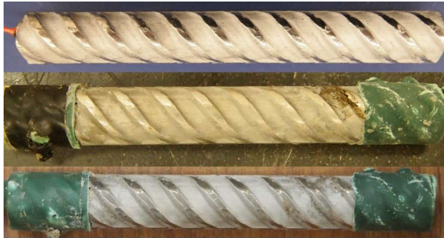
Figure C.1: RST 4-400 Batch – Corrosion Products on XM-28 AR 7.5. From top to bottom, a) original specimen, b) corrosion products on specimen upon removal from concrete, and c) pitting corrosion identification on a pickled specimen
