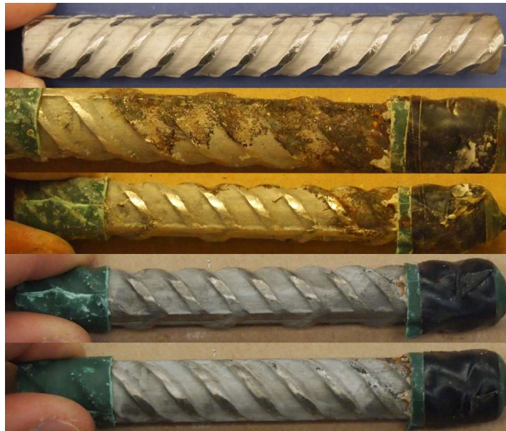
Figure C.30: 7.5-200 Batch – Corrosion Products on XM-28 AR 9.0. From top to bottom, a) original specimen, b) & c) corrosion products on the specimen upon removal from concrete, and d) & e) pitting corrosion identification on the pickled specimen. The slight staining at the top of the bar in a) is due to soldering flux.
