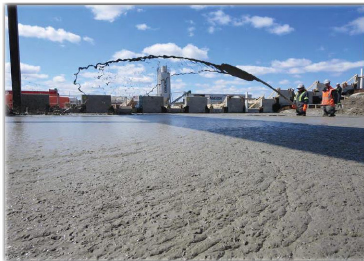
Figure 2-5: Lightweight Cellular Concrete being Placed with a Flexible Hose (Taylor et al., 2016)
