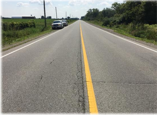
Longitudinal Cracking (centreline)
