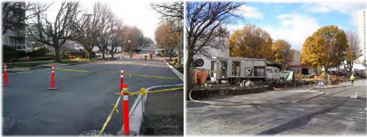
Figure 3-24: View Street and Vancouver Street Construction Process. Wet Mix Equipment (CEMATRIX)
