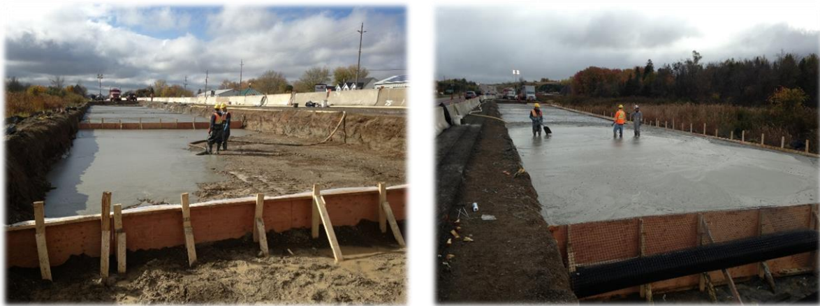
Figure 3-20: Highway 9 Construction Process (CEMATRIX)
