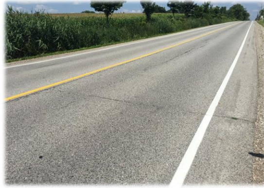
Transverse Cracking
