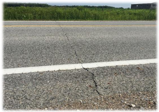
Transverse Cracking
