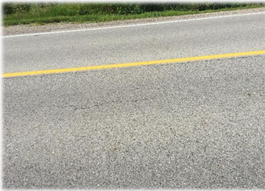
Longitudinal Cracking (centreline)
