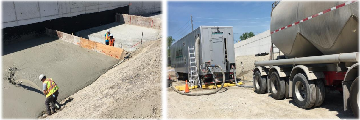
Figure 5-2: Construction Process. Toronto, May 2018
