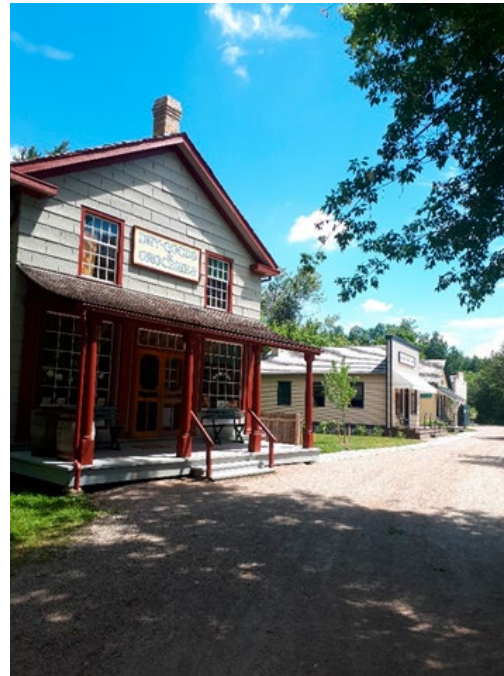
Figure 27.Several recreated edifications, shop, barber and bakery located in the heritage Village. each building allow the visitor a different experience.
