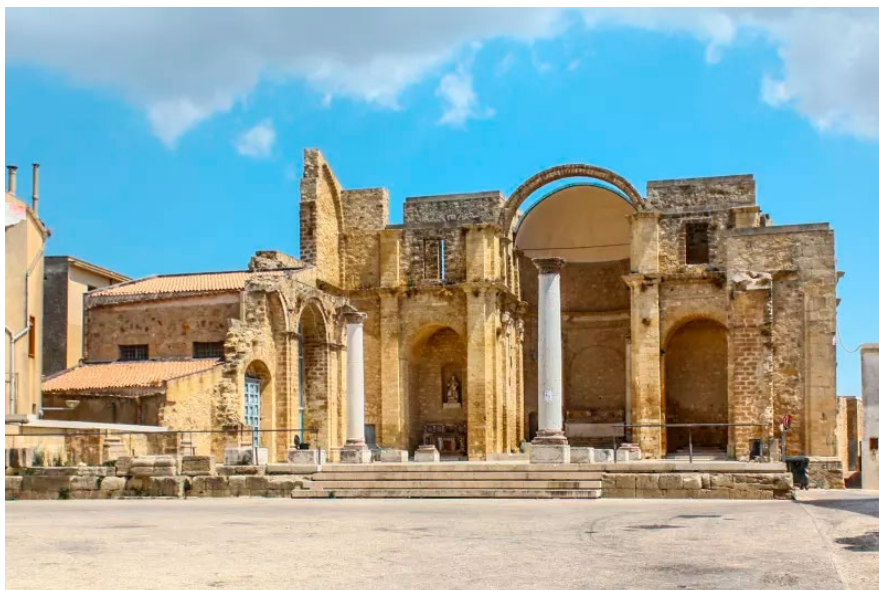
Figure 20. Piazza Alicia, Renewal project over the destroyed church dedicated to Our Lady Mother of the Angeal.
