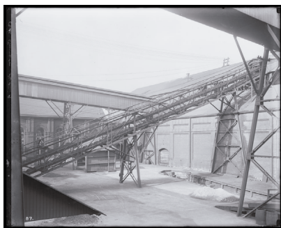
Figure 53. Coal Conveyors Station A.
