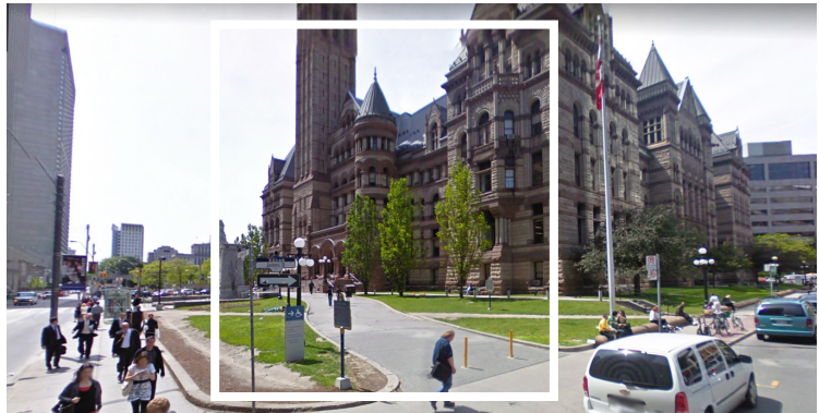
fig. 2.48 Corresponding existing view of the Projected Agora site from Google Map's Street View
