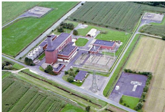
Figure 15 - Huntorf CAES plant [54]
