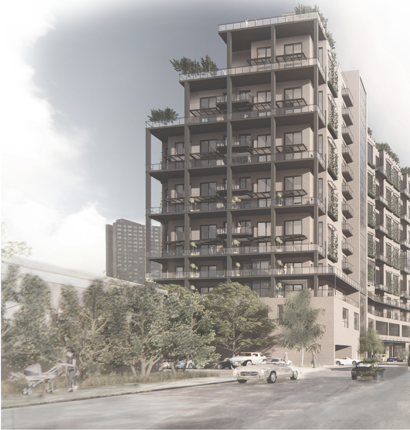
Fig 56. East Elevation Facing Bloor Street
