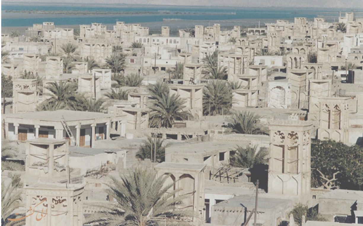
Fig 3. Port of Laft Overview, Qeshm Island
