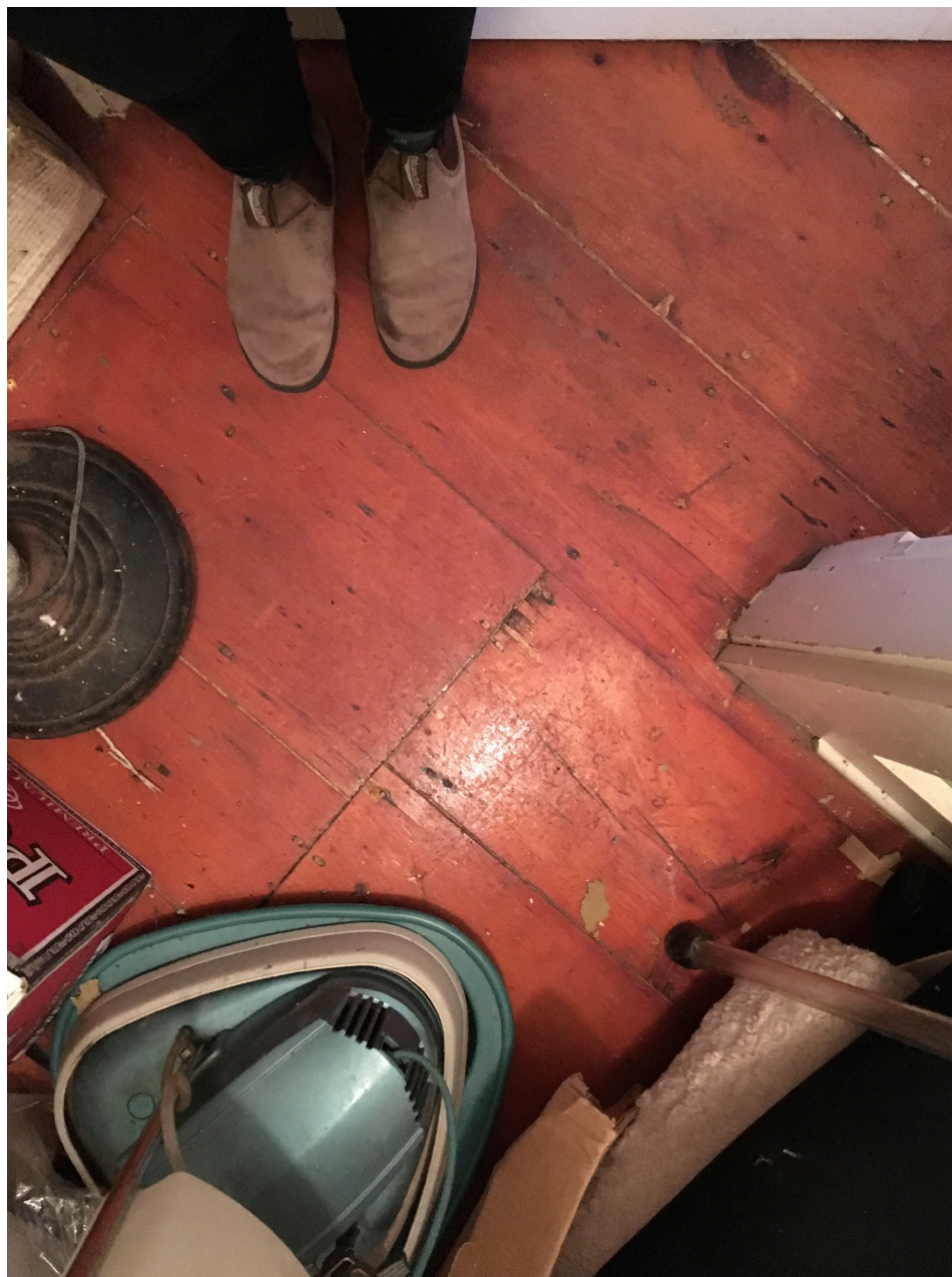
Figure 1-79 Evidence of the hatchway down to the false cellar
