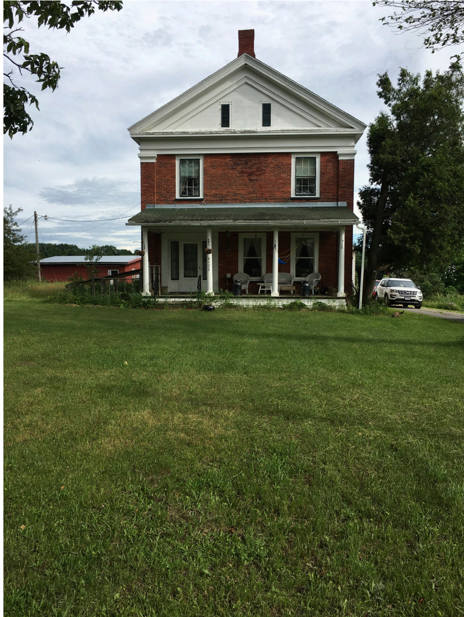
Figure 1-72 Front of the Coller House
