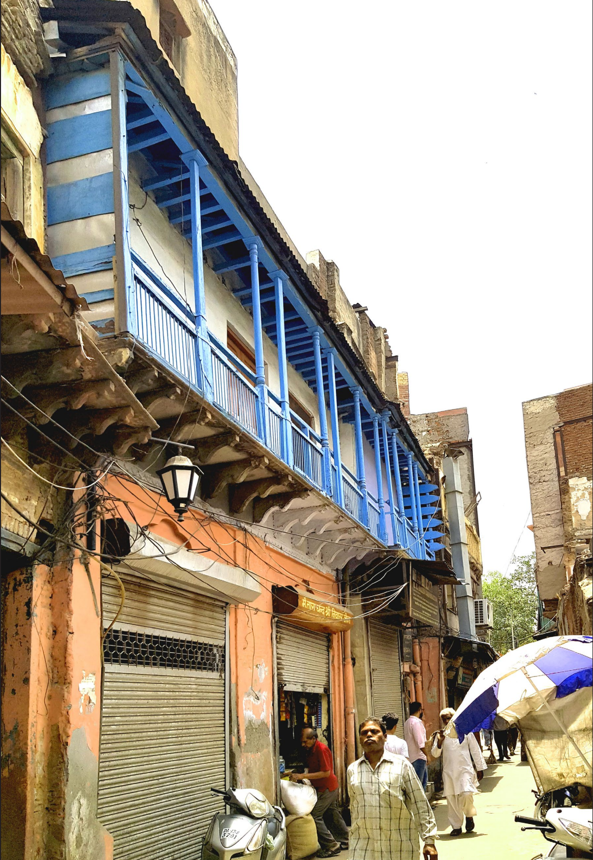
Figure 5.07 Common external corridor - use of vibrant colours
