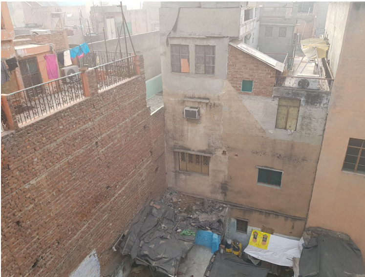
Figure 4.12 Collapsed Building site occupied by migrants
