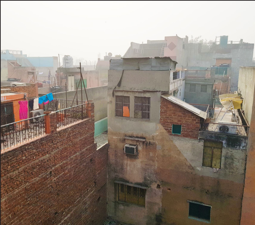
Figure 5.15 Houses looking into a collapsed hollow building site
