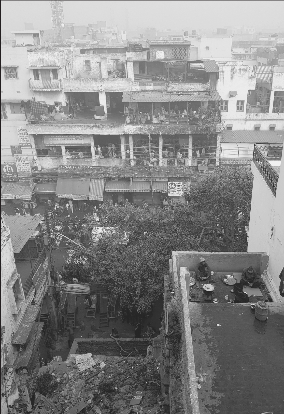
Figure 5.33 Collapsed building site
