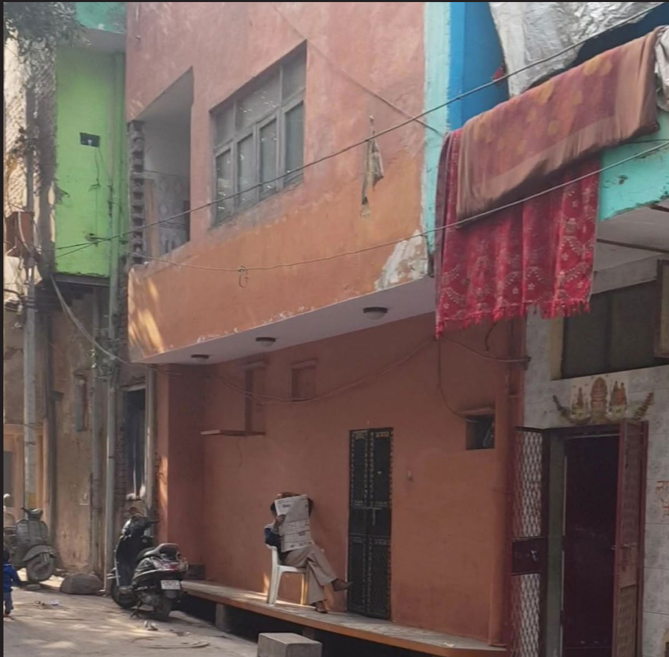
Figure 5.14 Raised plinth with water drainage passageway underneath
