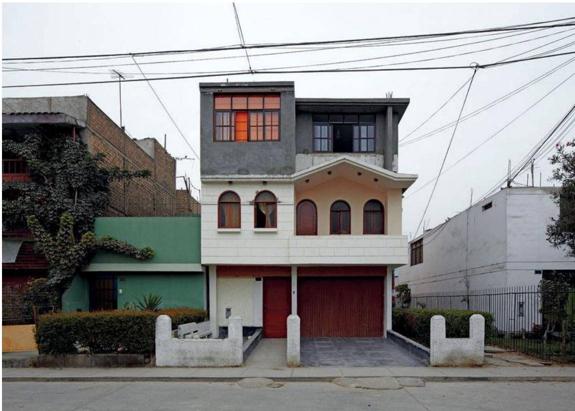
Figure 7.16 Charles Correa Scheme - Evolution overtime by addition of floor above the existing building
