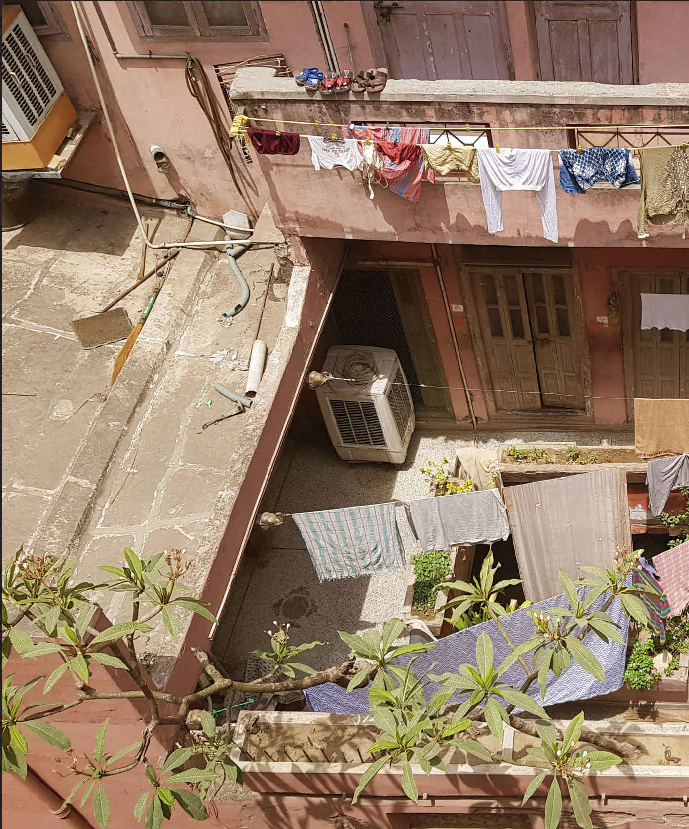
Figure 5.16 View from neighbours rooftop into an adjacent dwelling - depicts the two layers of the central courtyard. Original courtyard converted into a small light shaft.
