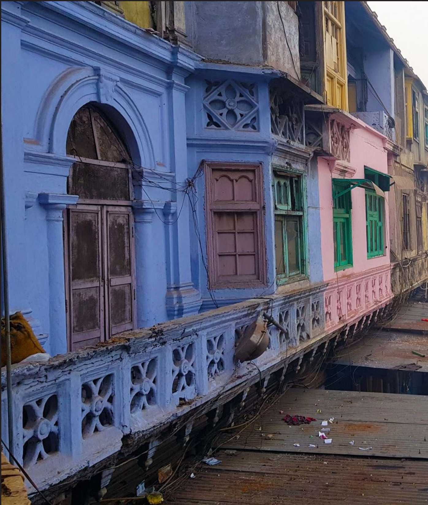
Figure 5.08 Gadodia Market - Retionship of the existing mansion with the now built up extensions and courtyard. Use of vibrant colours on the facades of the mansion.
