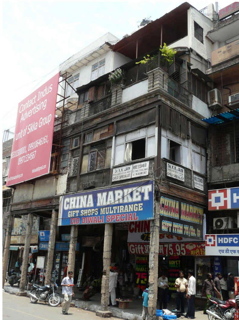
Figure 2.41 Photograph - Building on Chandni Chowk Road
