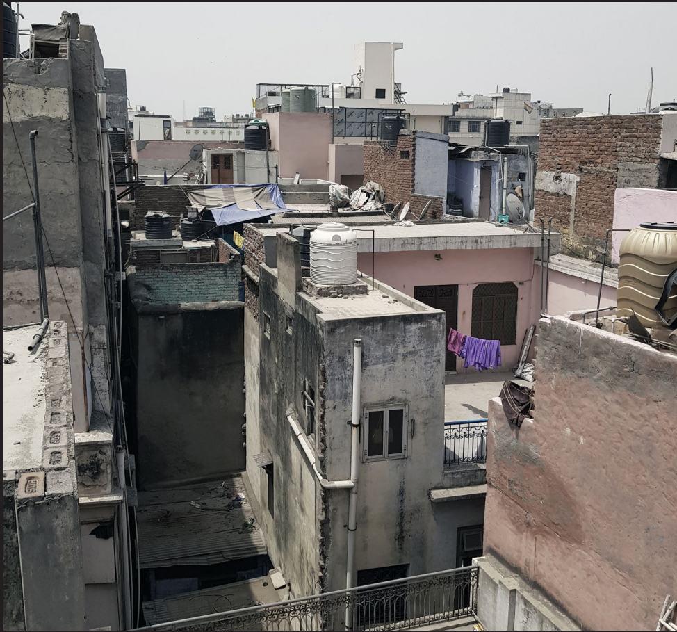
Figure 5.13 Small rooms constructed on rooftops
