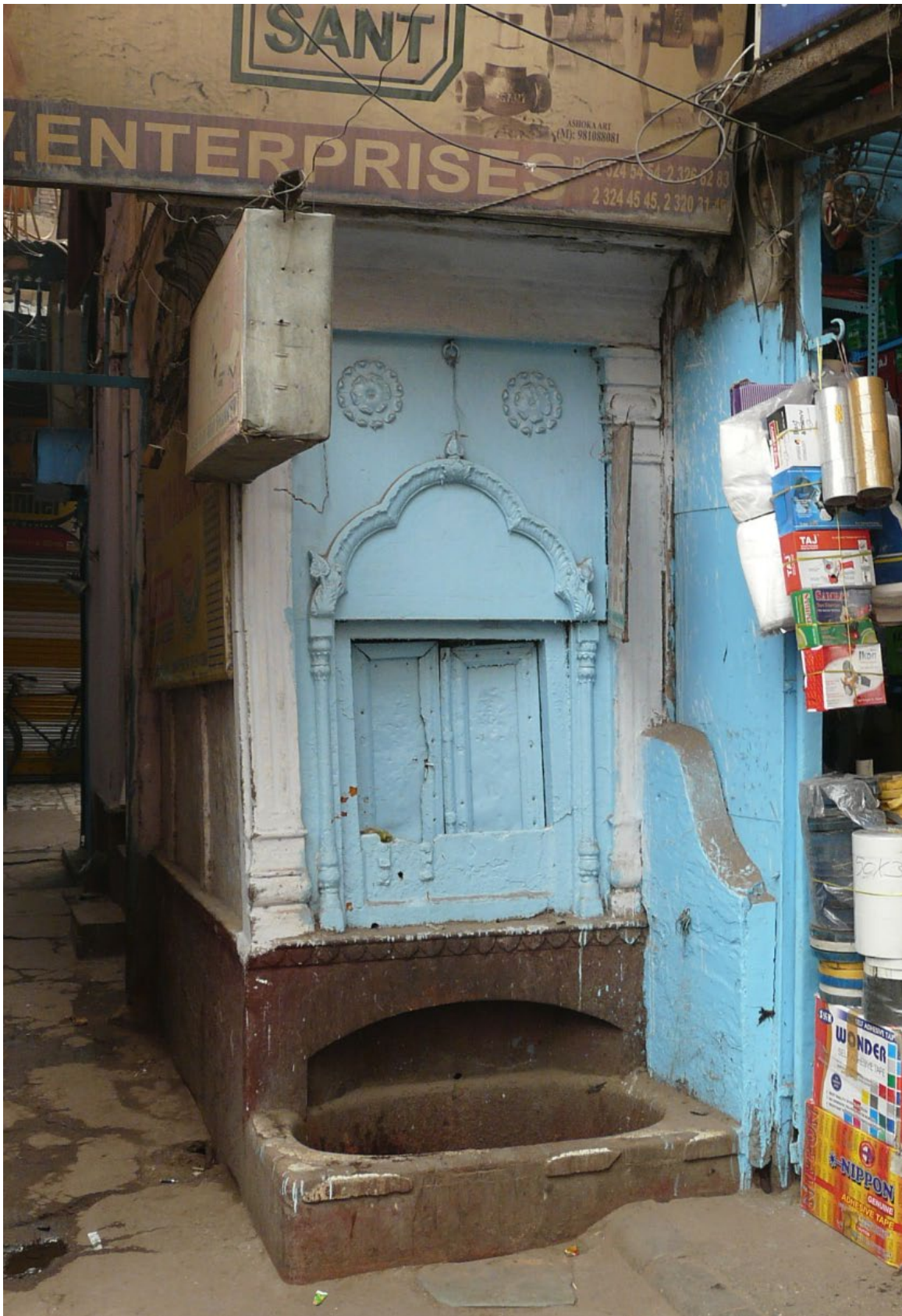
Figure 2.38 Pyau - Drinking water point
