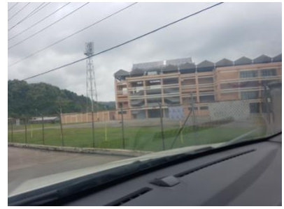
(Field Work Photos)
