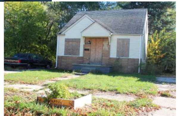
Figure 1.6: Abandoned Structures. Photo Montage by Author
