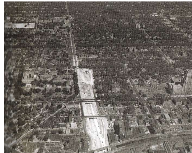
Figure 2.36 Aerial Photo showing construction of John C. Lodge Expressway (Hwy MI-10)
