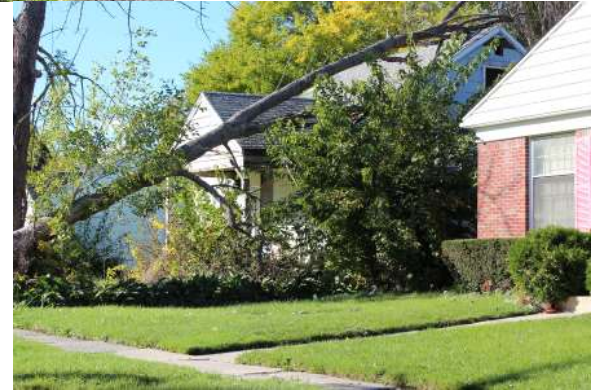
Figure 1.7: Structurally Damaged Structures. Photo Montage by Author
