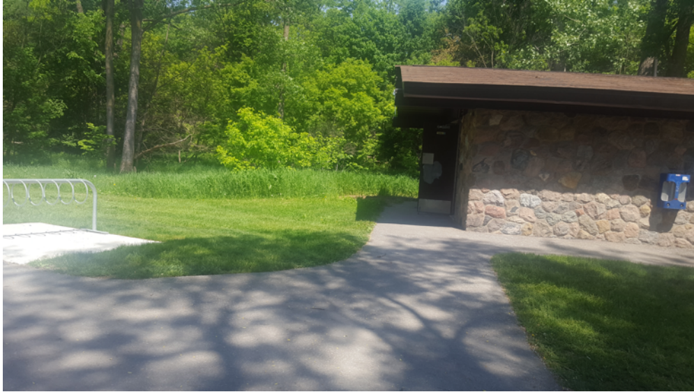
Image 7. Washroom and drinking fountain facility at Etienne Brulee Park
