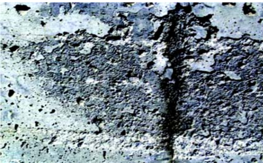
Figure 2-5: Concrete surface with medium spalling (ACI 201.1R-08)
