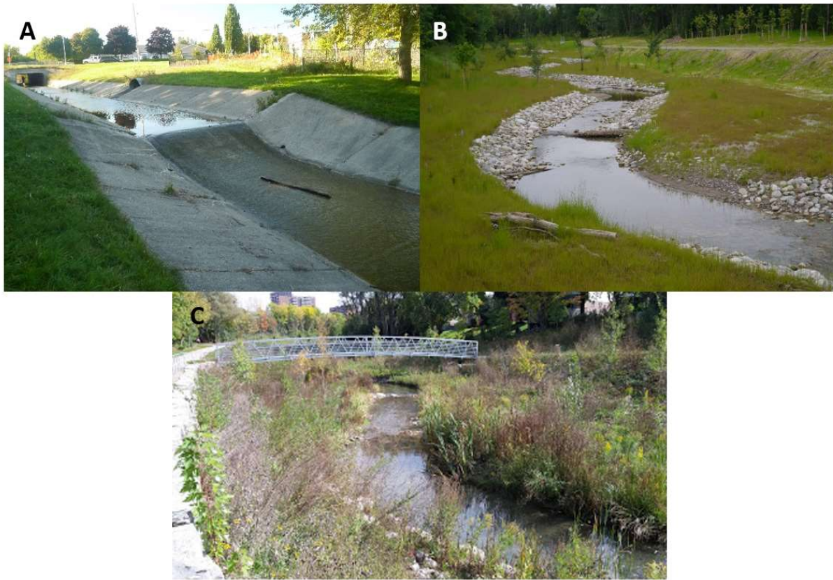
Figure 52: (A) Schneider Creek concrete channel (Krick, 2014) (B) Channel on June 19, 2015 after Fall 2014 construction (MacVicar, 2015) (C) Restored meandering channel (Muirhead, 2016)
