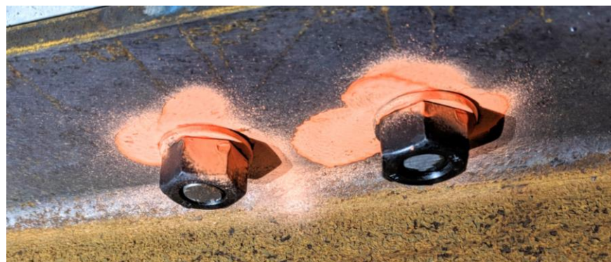
Figure 3-8: Spray painting of the embedded bolts for slip detection.
