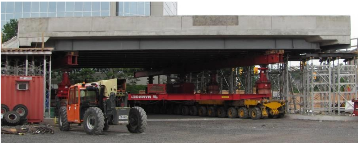
Figure 1-1: Rapid bridge replacement in Ottawa, Ontario.
