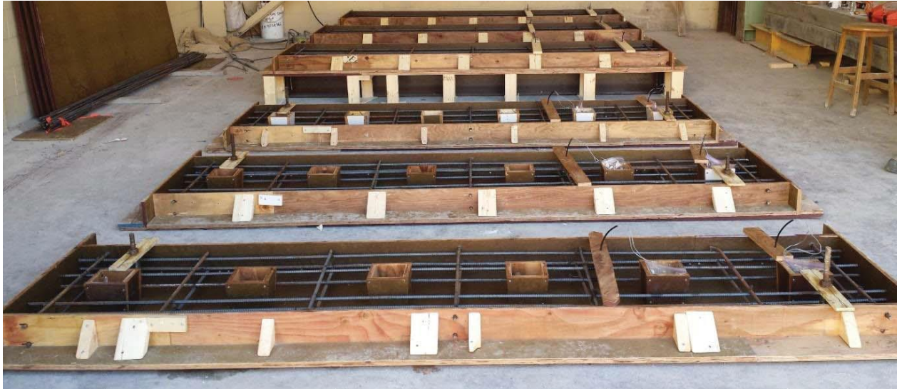
Figure 3-5: Precast formwork (foreground), and CIP formwork (background) for the stud specimens.
