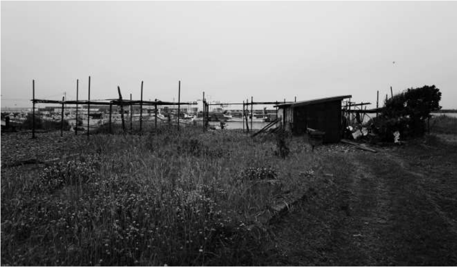
Figure 4.24 - Derelict structures common along the entirety of the town's edge.
