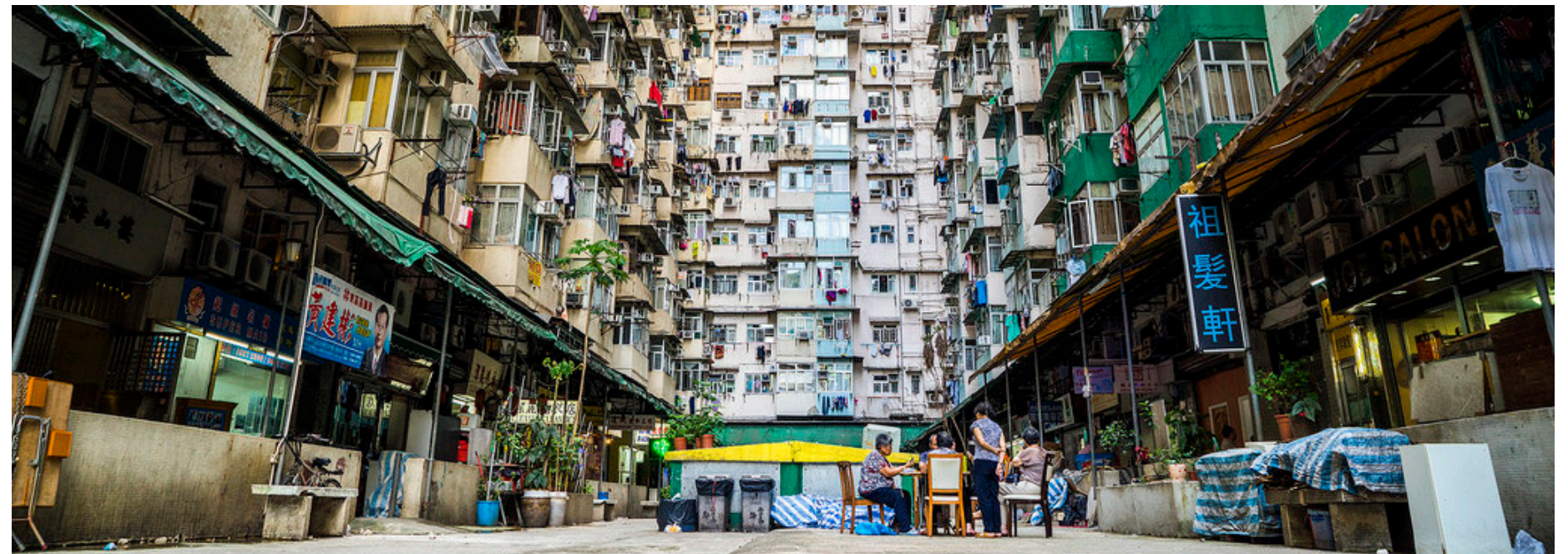
[Fig. 5.10] Typical alleyway
