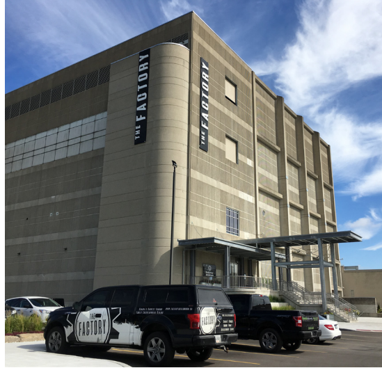
Figure 18 Photo of recently renovated rear of Kelloggs site in 2018. The indoor adventure park is just the first part of a larger development plan for the site.
