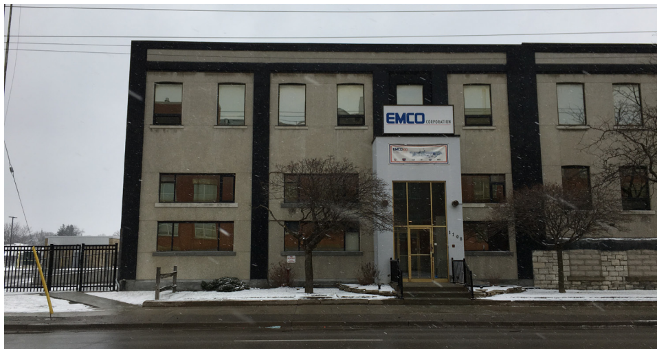
Figure 22 Photo of the exterior of EMCO in 2017.
