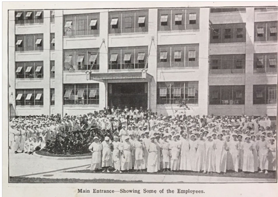
Figure 19 Photo of employees outside the McCormick factory showing the original condition of the exterior, Western Archives, Western University.
