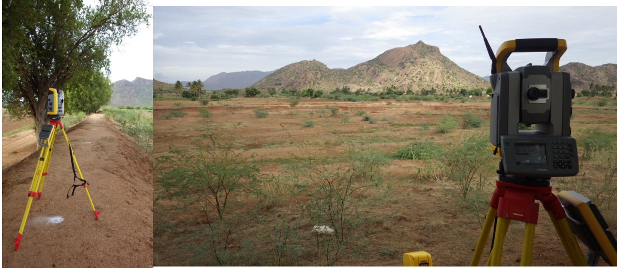
Figure A1: Topographic field survey in July 2016 using total station when tanks contained no water.
