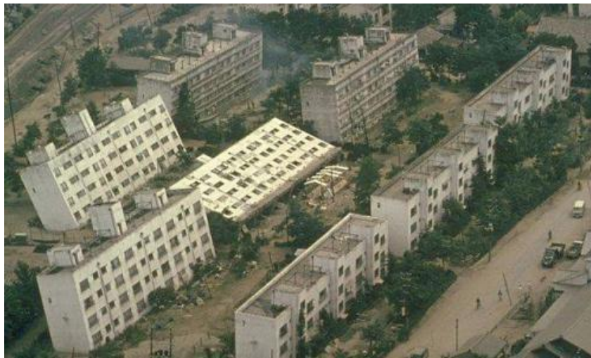
Figure 1.1 Liquefaction caused by the earthquake on buildings in Niigata, 1964 ( http://en.wikipedia.org/wiki/Soil_liquefaction#/media/File:Liquefaction_at_Niigata.JPG )
