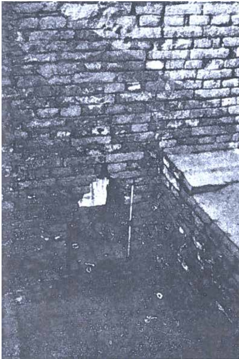
Fig. 68 — A small opening for a drain, disposal chute, and ventilation.
