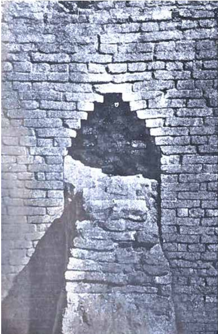
Fig. 67 — A primitive arch opening for a drainage chute
