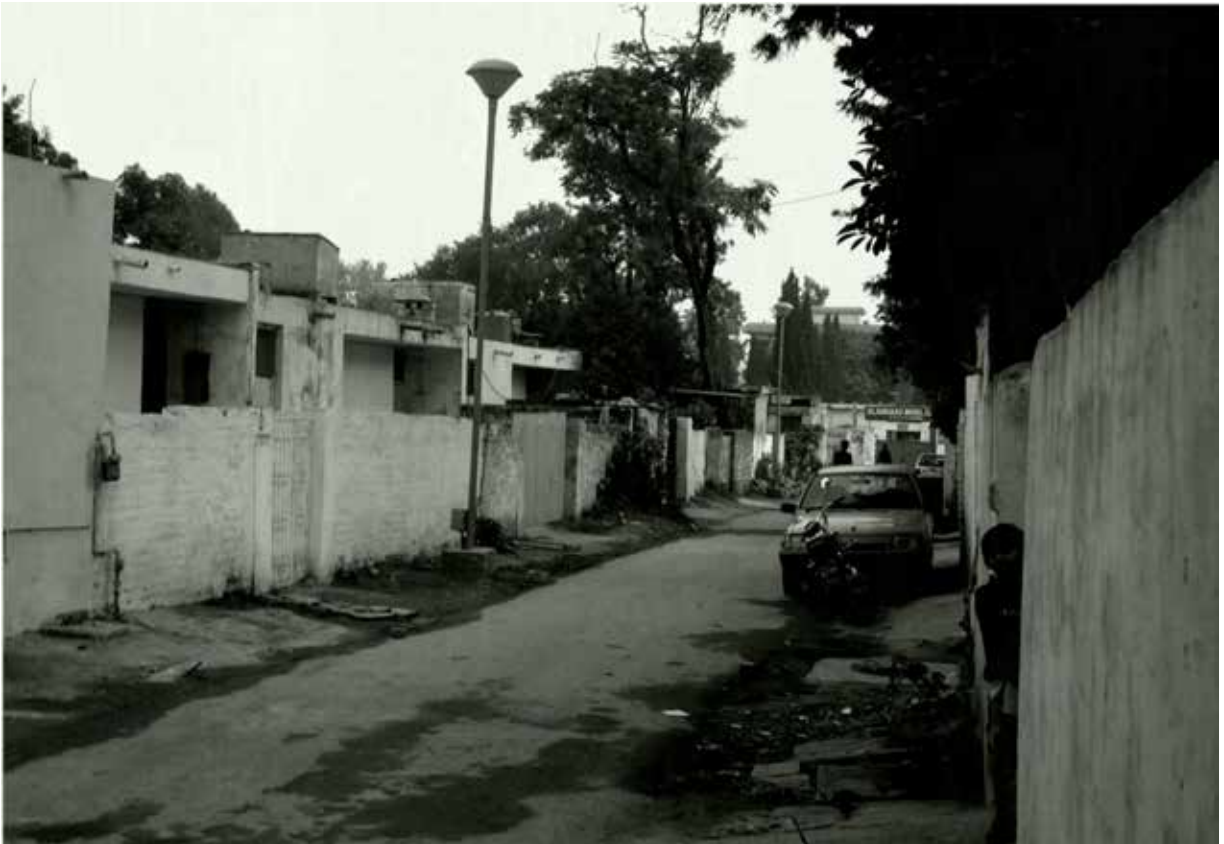
Fig. 50 —Original low-income housing from Doxiadis' plan for Islamabad in its current state.
