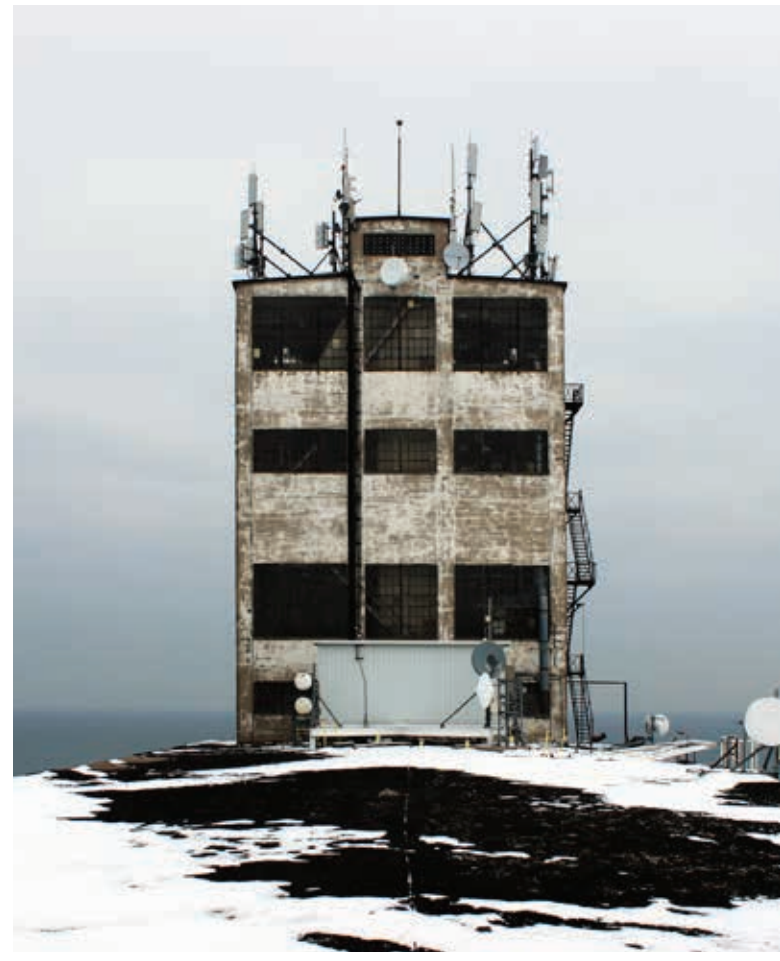
Figure 1.9 [Above] Head House Tower of the Collingwood Terminals from the roof of the distributing floor. Note the ad-hoc composition of the various telecommunications arrays.
