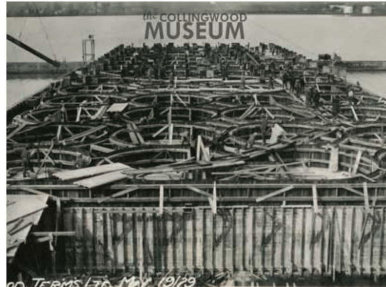
Figure 2.17 [Left] May 17, 1929. Concrete slip forms are placed atop the storage bin floor-slab. Each storage vessel receives two openings for grain passage to the work floor below. Note the further division within the central foreground cylindrical formwork, creating vertical chases to house the grain elevator belts.
