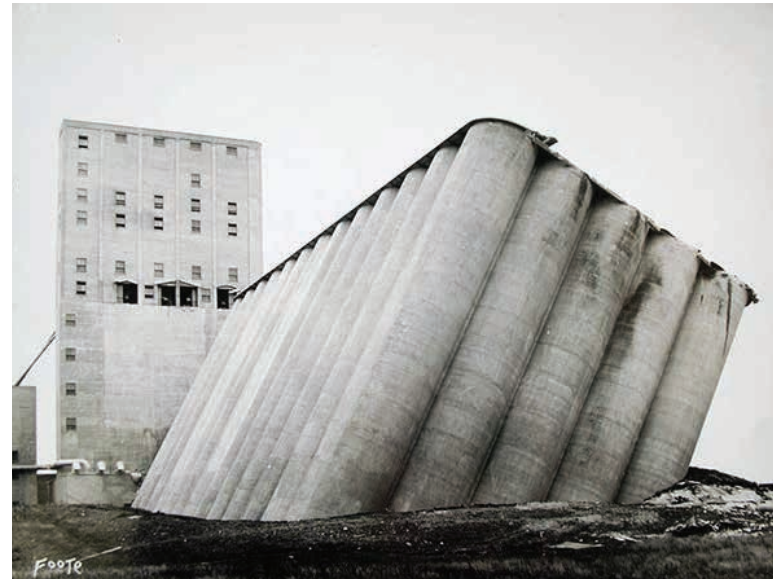
Figure 2.8 Soil bearing failure at the newly constructed Transcona Grain Elevator, circa 1913. The robust construction defied the stresses of the collapsed foundations and the monolithic storage bins were righted without incident. The elevator remained in use throughout much of the 20 th century.
