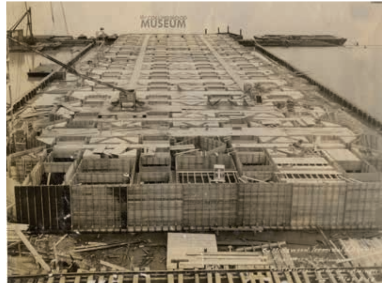
Figure 2.14 [Left] Work Floor formwork, with conveyor hallways oriented under the centreline of the storage bins above.
