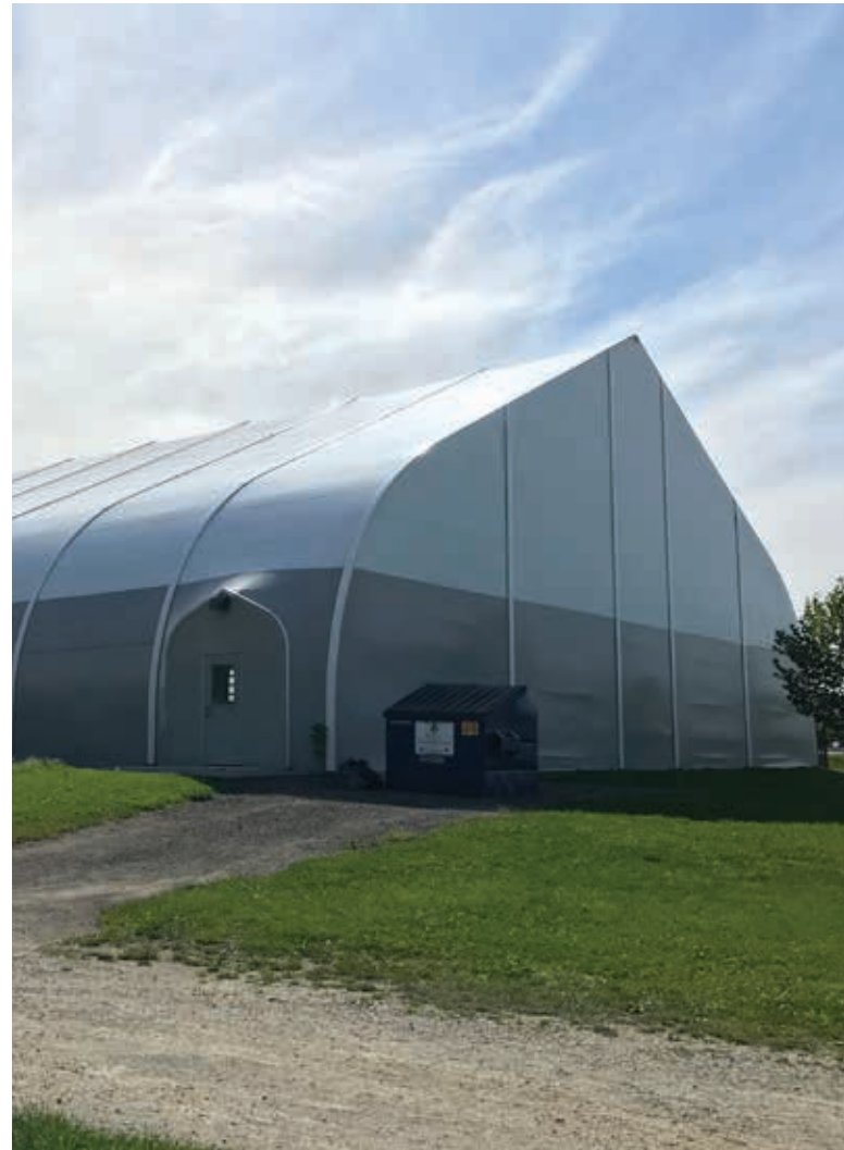
Figure 2.38 [Right] Centennial Pool, 2018. $12.4 million does not include landscaping or well-placed services. Sags and rips are prevalent in the enclosure membrane.
