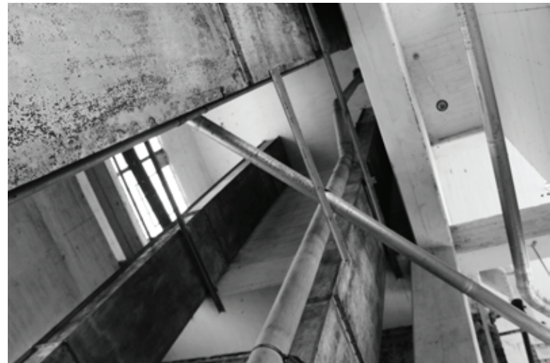
Figure 5.44 [Opposite] Encased grain elevator between hoppers and holding tanks.
