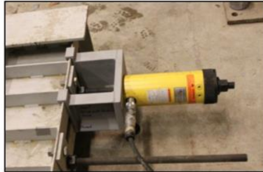
b) Jack installed on the threaded
