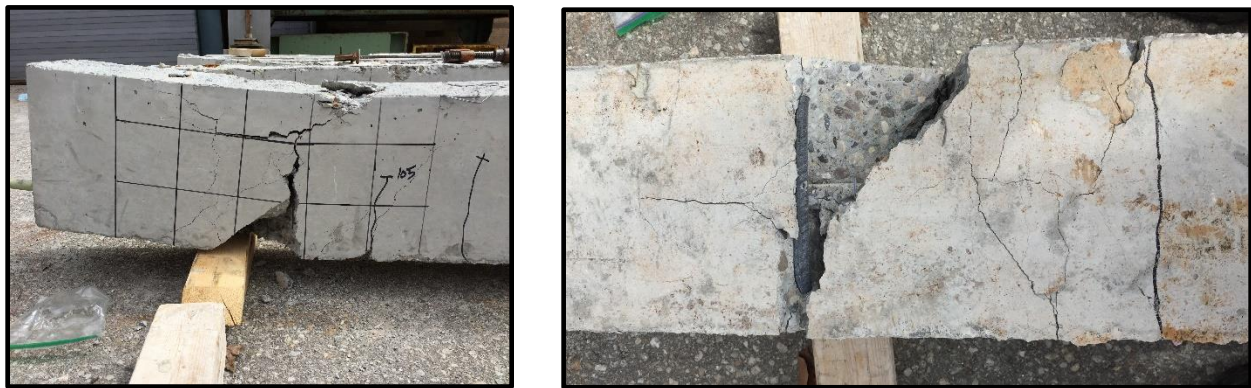
Figure 5.31: Typical bond failure for beam reinforced with sand coated GFRP bar
