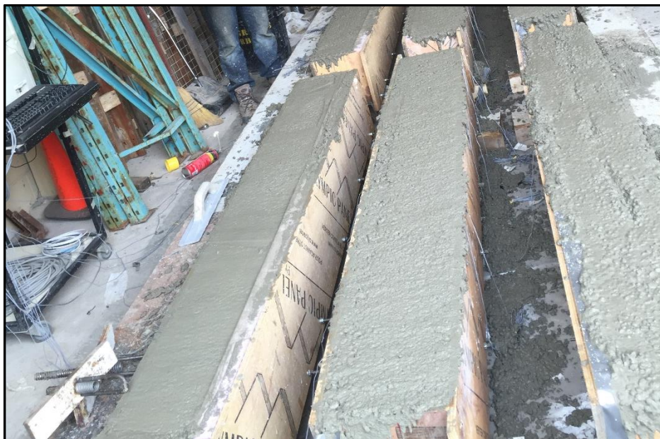
Figure 3.8 Formwork filled with concrete
