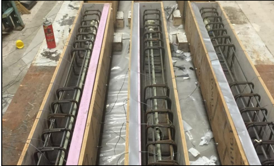
Figure 3.7 Steel cage inside the form placed on the prestressing bed
