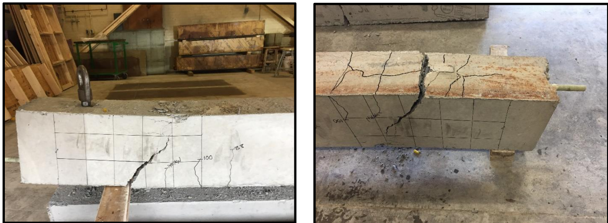
Figure 5.17 typical bond failure
