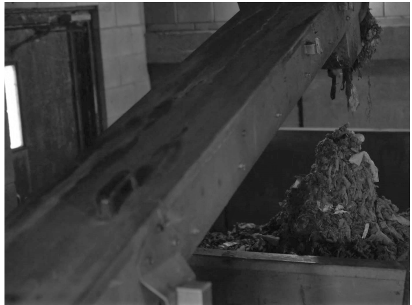
Figure.19 Filtration Process: Removal of large solids
