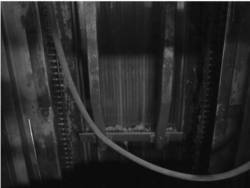
Figure.18 Filtration Process: Grit Channel
