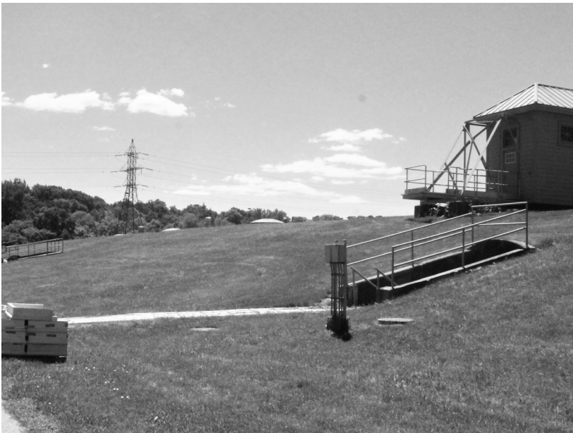
Figure.28 Filtration Process: Entrance to underground digestors
