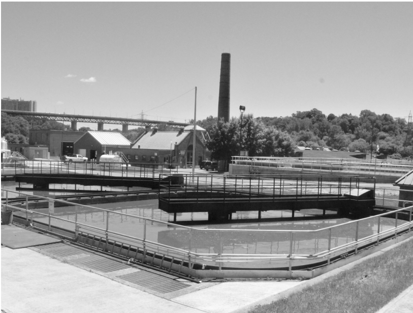
Figure.21 Filtration Process: Primary Clarification Tanks
