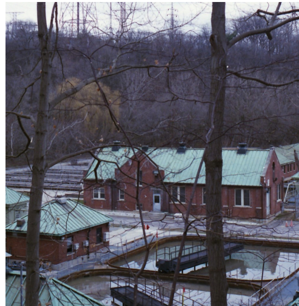
Figure.13 NTWWTP from the trail
