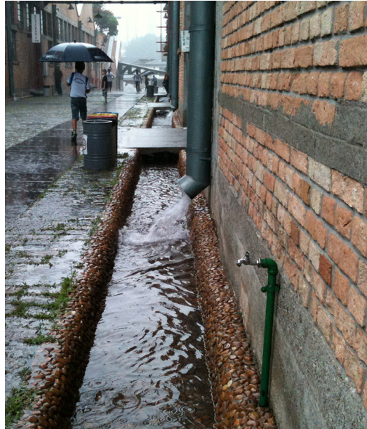
Figure.44 SESC Pompica rain drainage, 1986, Lina Bo Bardi
