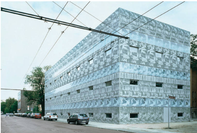
FIG 2.9 EBERSWALDE TECHNICAL SCHOOL LIBRARY BY HERZOG & DE MEURON, 1999.
