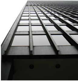
FIG 1.5 SEAGRAM BUILDING (LOOKING UP AT THE ORNAMENTAL STEEL MEMBERS) BY LUDWIG MIES VAN DER ROHE, 1958.
