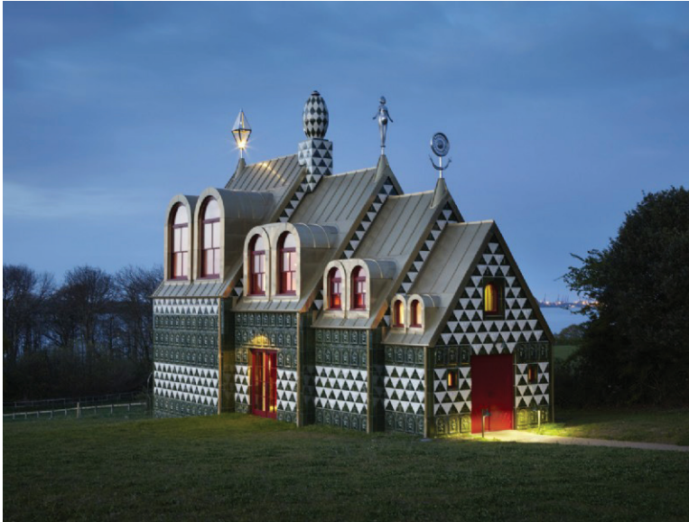
FIG 4.2 A HOUSE FOR ESSEX - A COLLABORATION BETWEEN ARTIST GRAYSON PERRY AND FAT ARCHITECTURE, 2014. VIEW OF THE SOUTH ENTRANCE.
