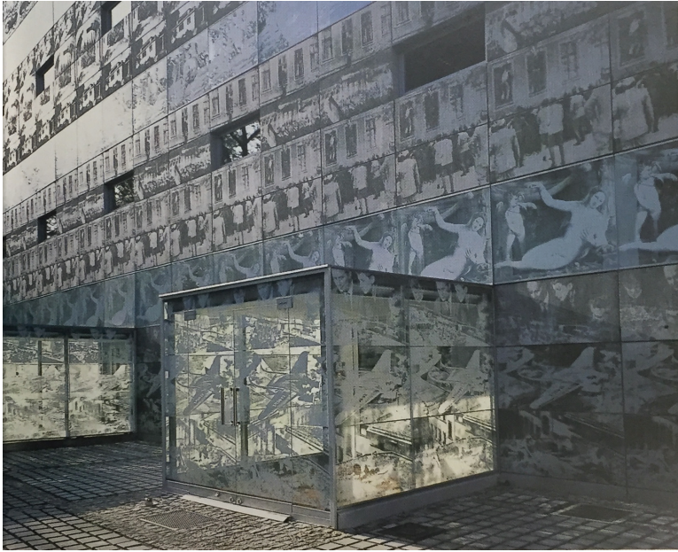
FIG 3.8 EBERSWALDE TECHNICAL SCHOOL LIBRARY BY HERZOG & DE MEURON, 1999.
