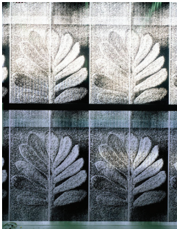
FIG 3.7 PRINTED PANELS ARICOLA-EUROPE STORAGE AND PRODUCTION BUILDING BY HERZOG & DE MEURON ARCHITECTS, 1993.
