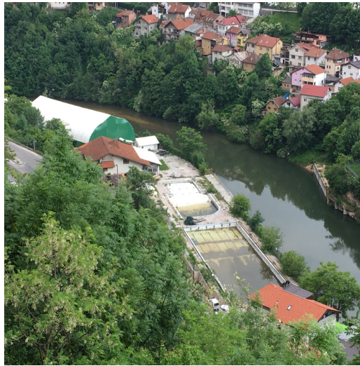
Figure 3.32 Point 2 - The Bentbaša Pools The heart of the project
