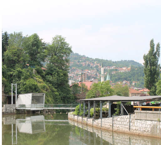
Figure 3.3 Existing 'Tekke' Ruin Canopy, 2018
