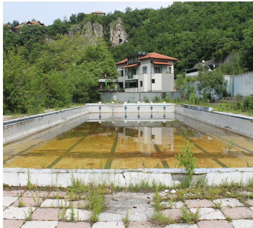
Figure 3.6 Existing Bentbaša Pools, 2018
