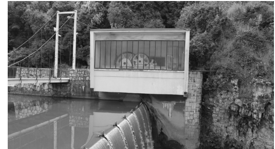
Figure 1.27 Modernized Pools at Bentbaša Figure 1.28 Bentbaša Dam, Gearbox & Pedestrian Bridge
