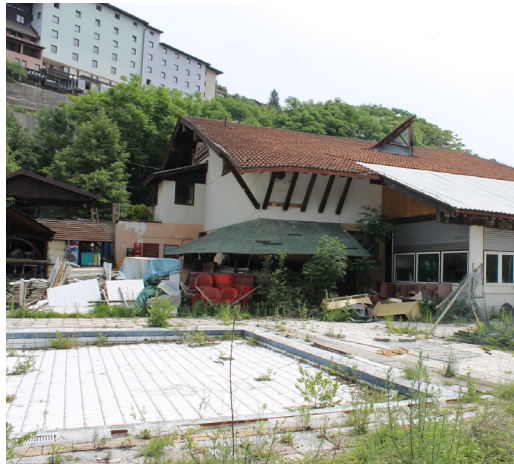
Figure 3.9 Existing Bentbaša Storage Structures, 2018
