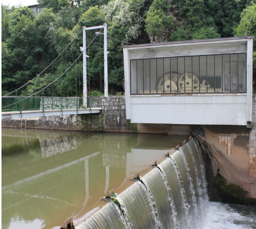
Figure 3.2 Existing Bentbaša Dam & Gearbox, 2018
